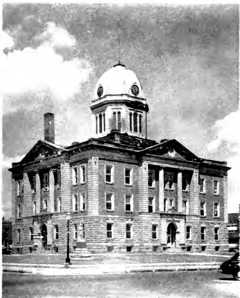
THE COURTHOUSE OF MOULTRIE COUNTY Sullivan, Illinois
