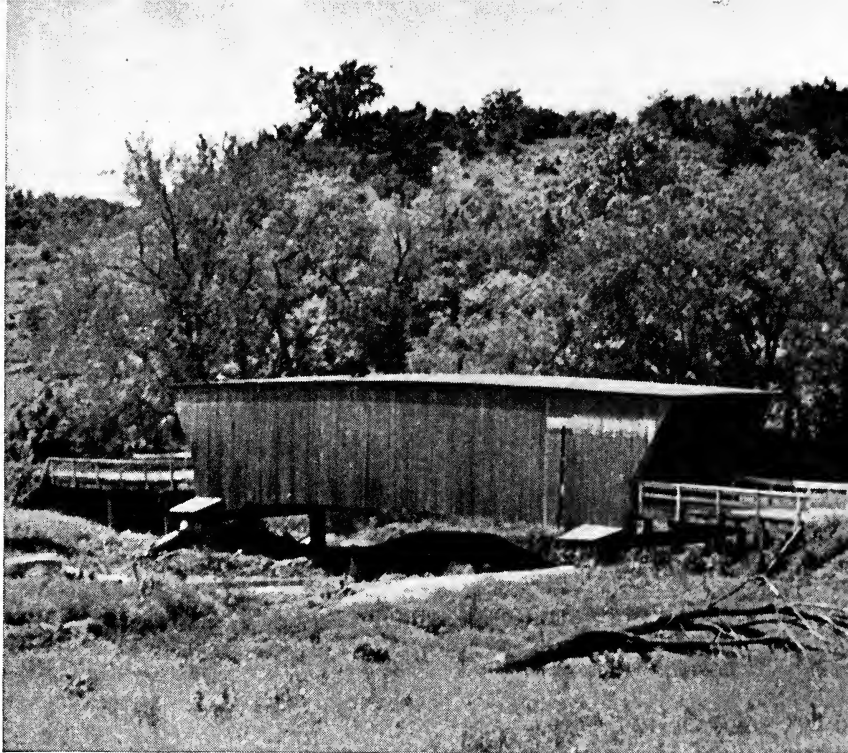
COVERED BRIDGE, MADISON COUNTY
