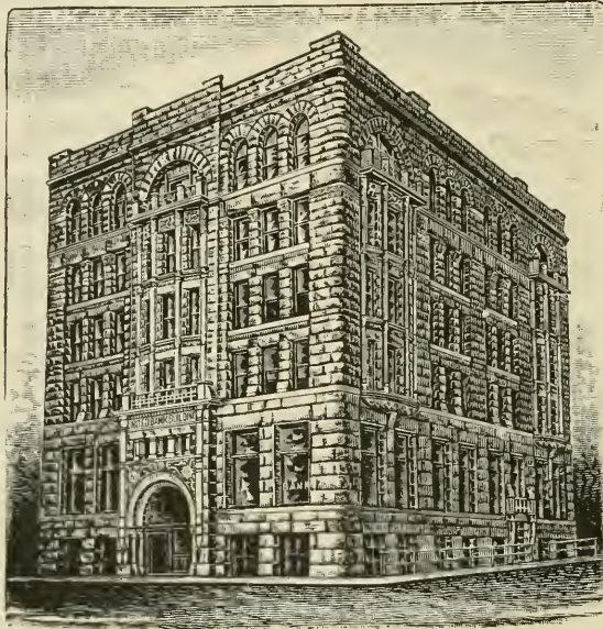
UNITED BANK BUILDING, SIOUX CITY.
