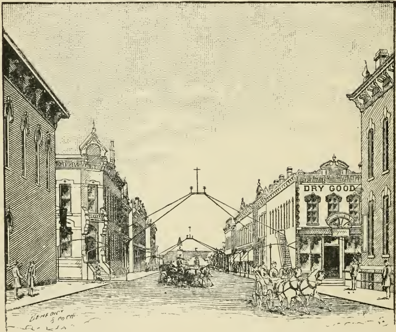
SCENE LOOKING WEST ON MONTGOMERY STREET.
