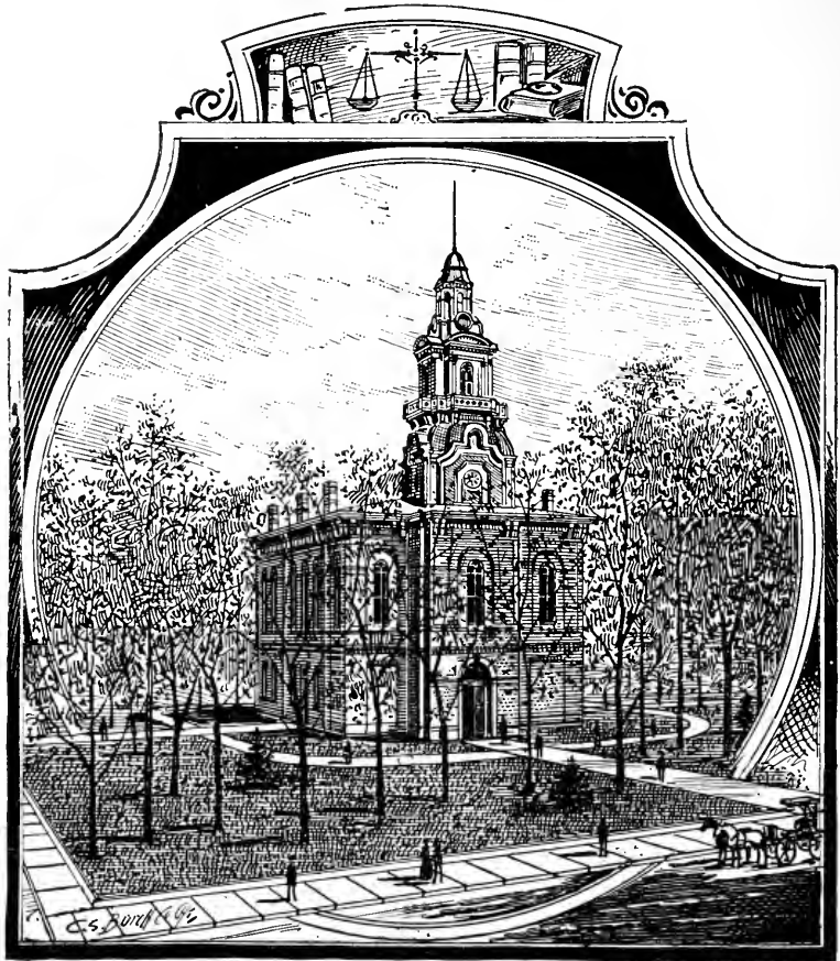
COURT-HOUSE AT CENTREVILLE.
