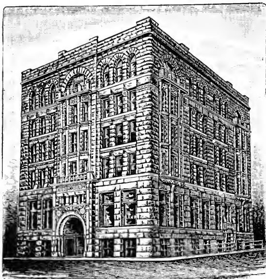
UNITED BANK BUILDING, SIOUX CITY.
