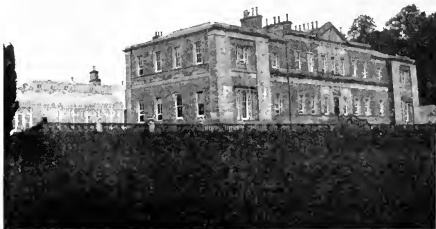
Agricultural Station, Ballyhaise, Co. Cavan
