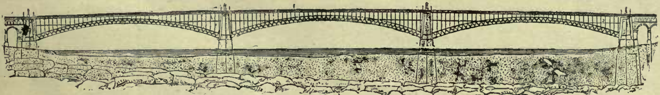
ST. LOUIS AND ILLINOIS BRIDGE. (No. 19)
