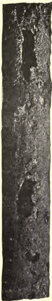
FIG. 29.—Wrought-iron pipe corroded in the soil.
