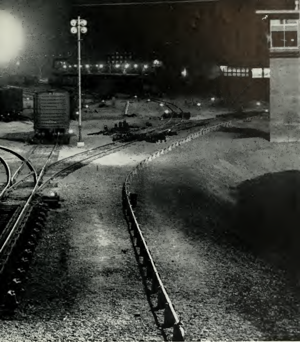
23 Armourdale (Kansas City, Kansas) automatically-controlled hump yard, can handle classification of 4,000 cars daily.
