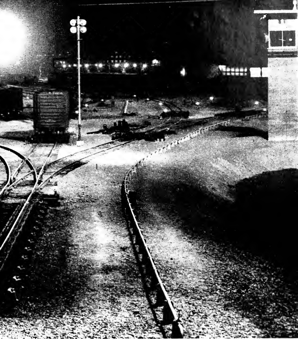
25 Armourdale (Kansas City, Kansas) automatically-controlled hump yard can handle classification of 4,000 cars daily.
