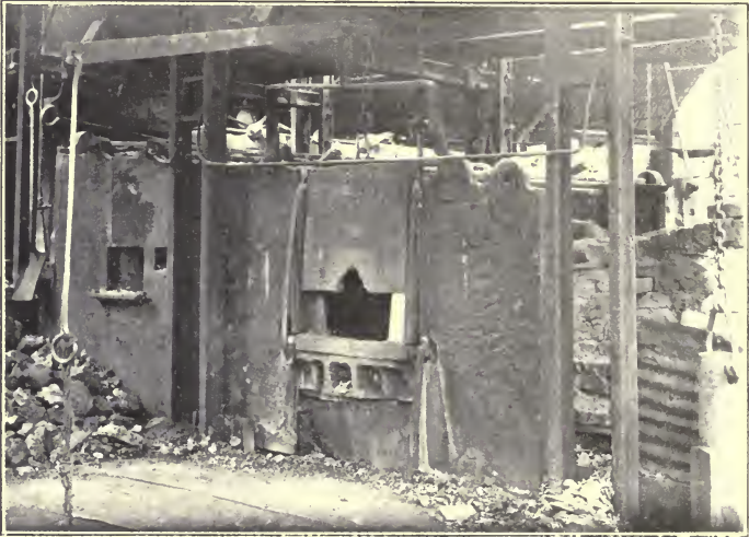
FIG. 23.—Working Side of Puddling Furnace.
