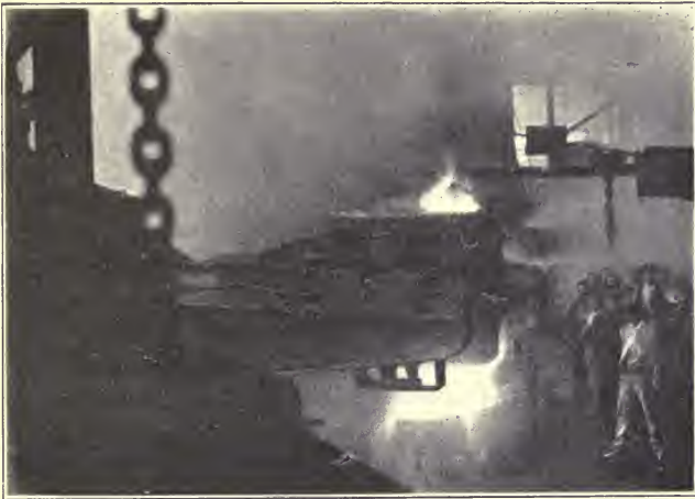
FIG. 36.—Casting Basic Steel at Spring Vale Works.
