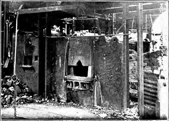
FIG. 23.—Working Side of Puddling Furnace.
