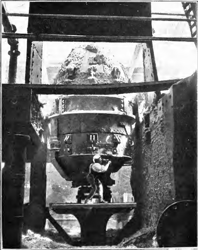
FIG. 34.—Bessemer Converter in Position.
