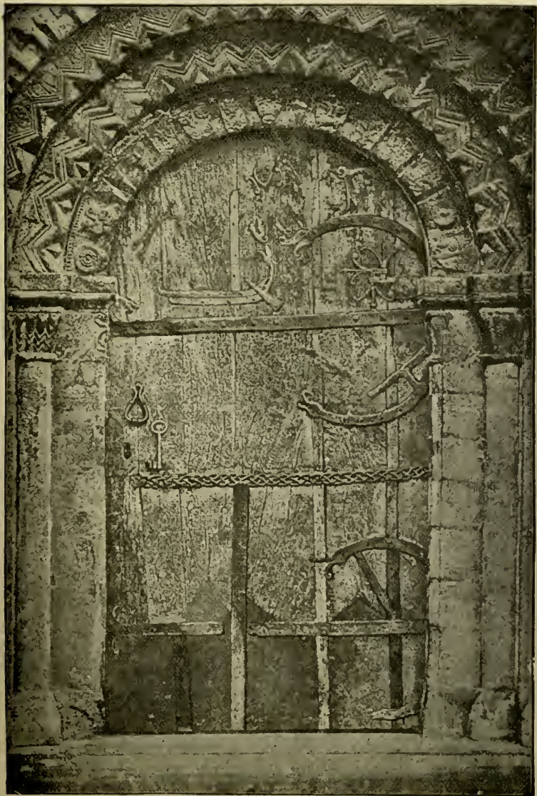
FIG. 17.—Hinges, etc., at Stillingfleet Church.
