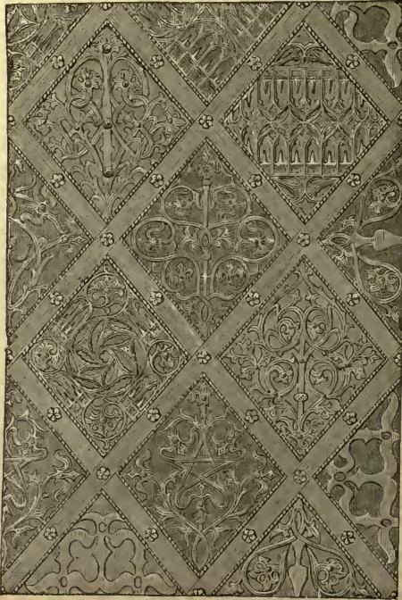
FIG. 54.—Part of door in the Priory of Bruck, with pierced and embossed ironwork.
