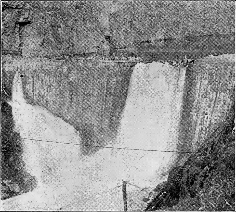
THE LA GRANGE DAM NEARLY COMPLETED, TUOLUMNE RIVER, CAL.
