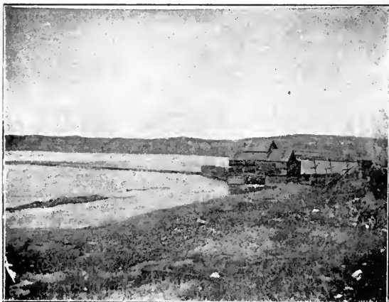
VIEW OF PLANT, LOOKING UP STREAM.
