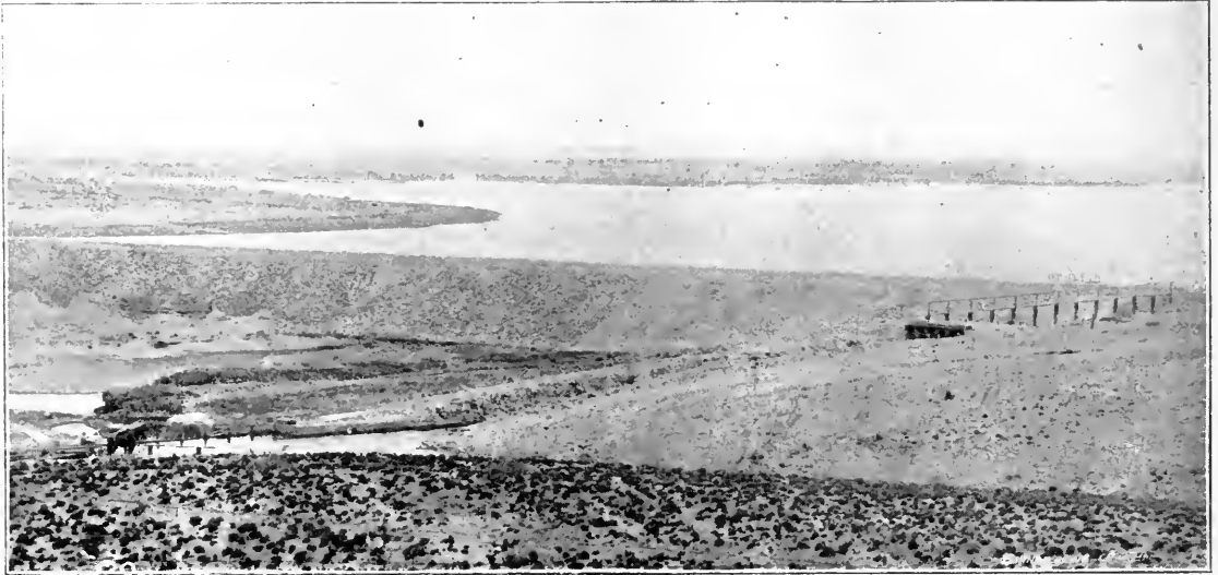
EDDY DISTRIBUTING RESERVOIR, PECOS VALLEY SYSTEM.
