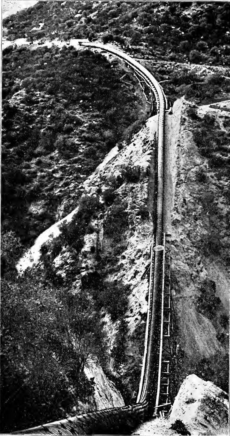
SIPHON PIPE, BEAR VALLEY SYSTEM.
