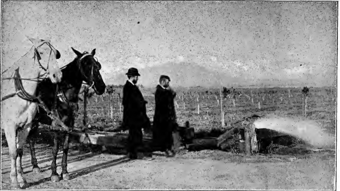
YOUNG ORANGE GROVE. HYDRANT CONNECTED WITH IRRIGATION SYSTEM. VAL VERDE TRACT.
