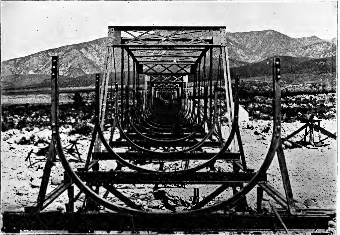
BUILDING A FLUME ON THE BEAR VALLEY SYSTEM.
