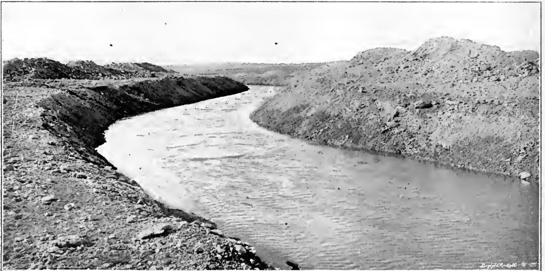
VIEW OF MAIN CANAL, PECOS VALLEY IRRIGATION SYSTEM.
