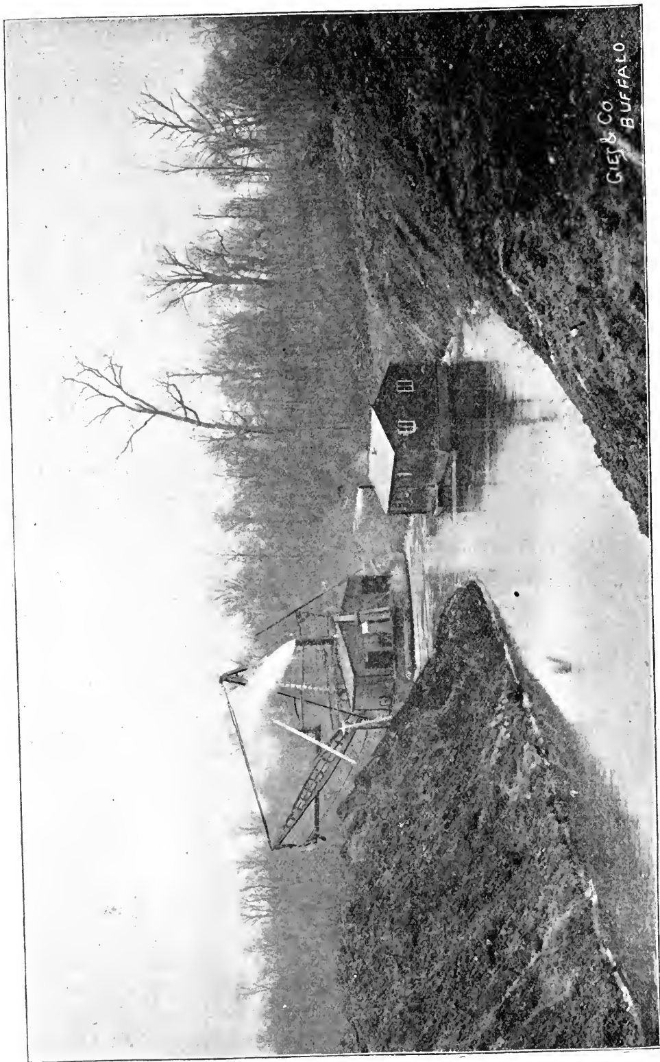
BARNHART DREDGE AT WORK BUILDING A DITCH.
