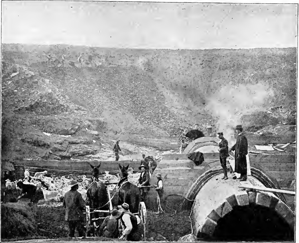
GOATS PUDDLING THE EARTHWORK OF A DAM IN NEW MEXICO.
