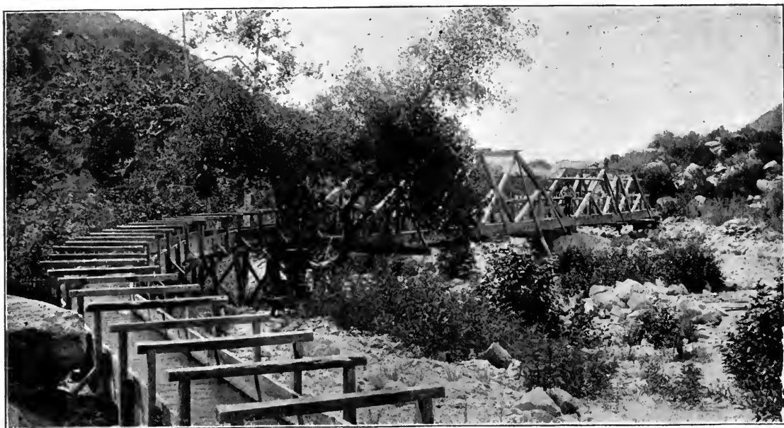
A VIEW OF THE FLUME LINE OF THE HEMET LAND COMPANY.
