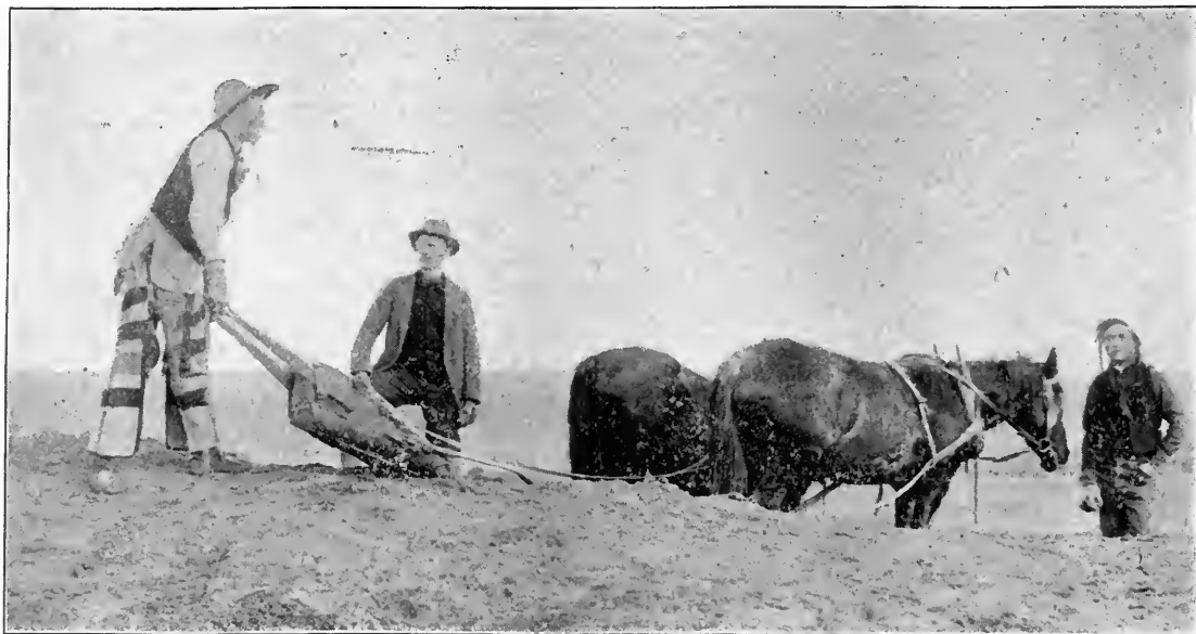
THE FIRST LESSON IN CANAL BUILDING ON THE CROW AGENCY, UNDER THE INSTRUCTION OF WALTER H. GRAVES.*
