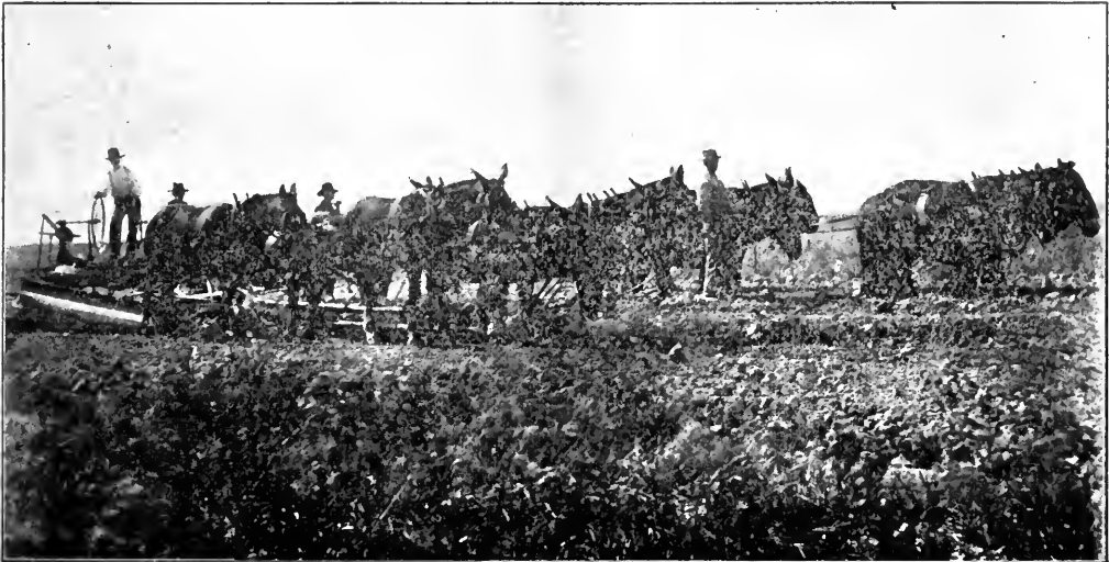
DITCHING MACHINE AT WORK.
