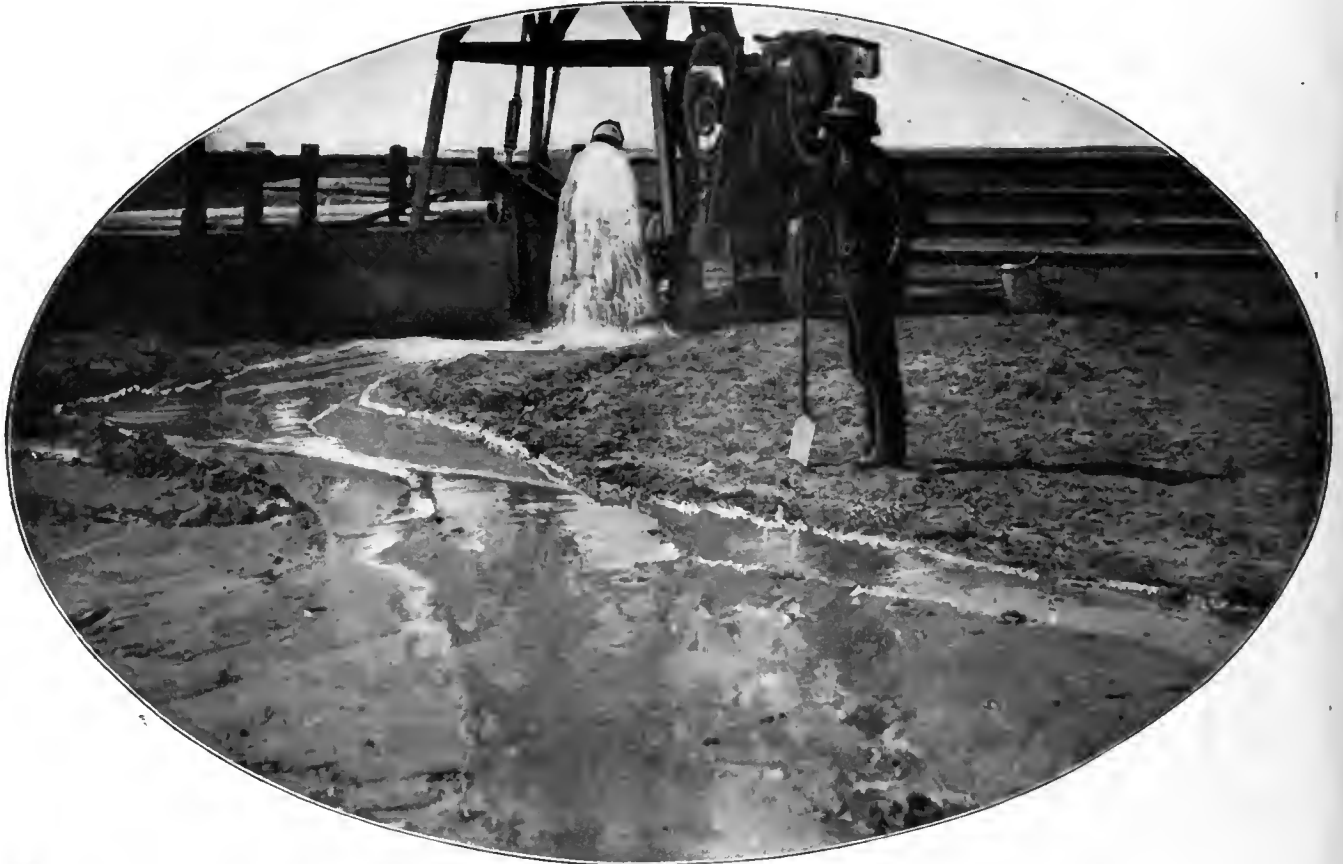
CENTRIFUGAL PUMP AND GASOLINE ENGINE IRRIGATION OUTFIT.
