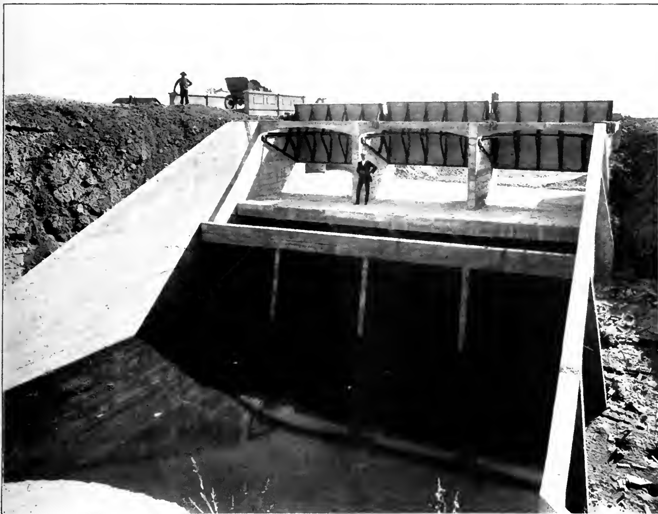
Division Gate No. 1—Kicking Bird Canal. Note the solid appearance of the concrete work and the patent gates which are also made of reinforced concrete.
