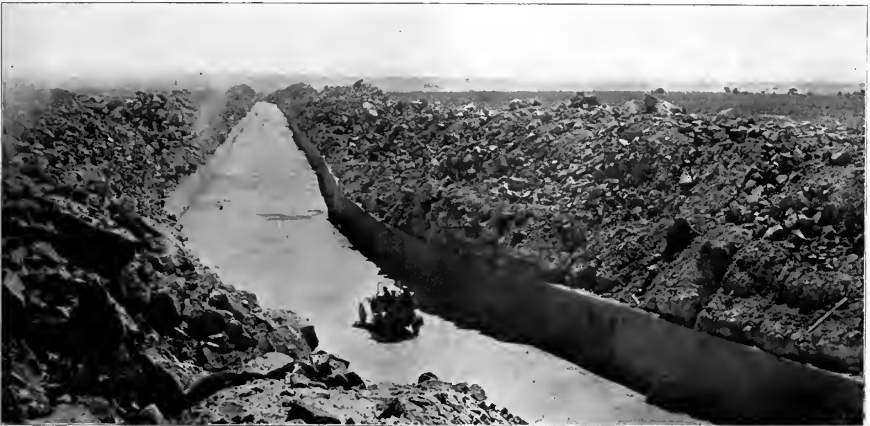
Main irrigation canal, Twin Falls North Side tract, showing heavy rock cut and concrete lining. This canal will supply water for more than 200,000 acres of land.
