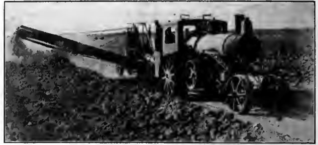
Pulling Reversible Excavator on Irrigation Work.
