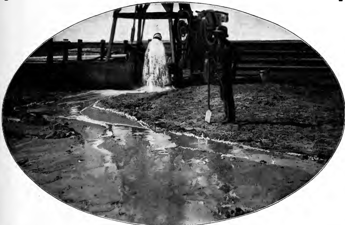
CENTRIFUGAL PUMP AND GASOLINE ENGINE IRRIGATION OUTFIT.
