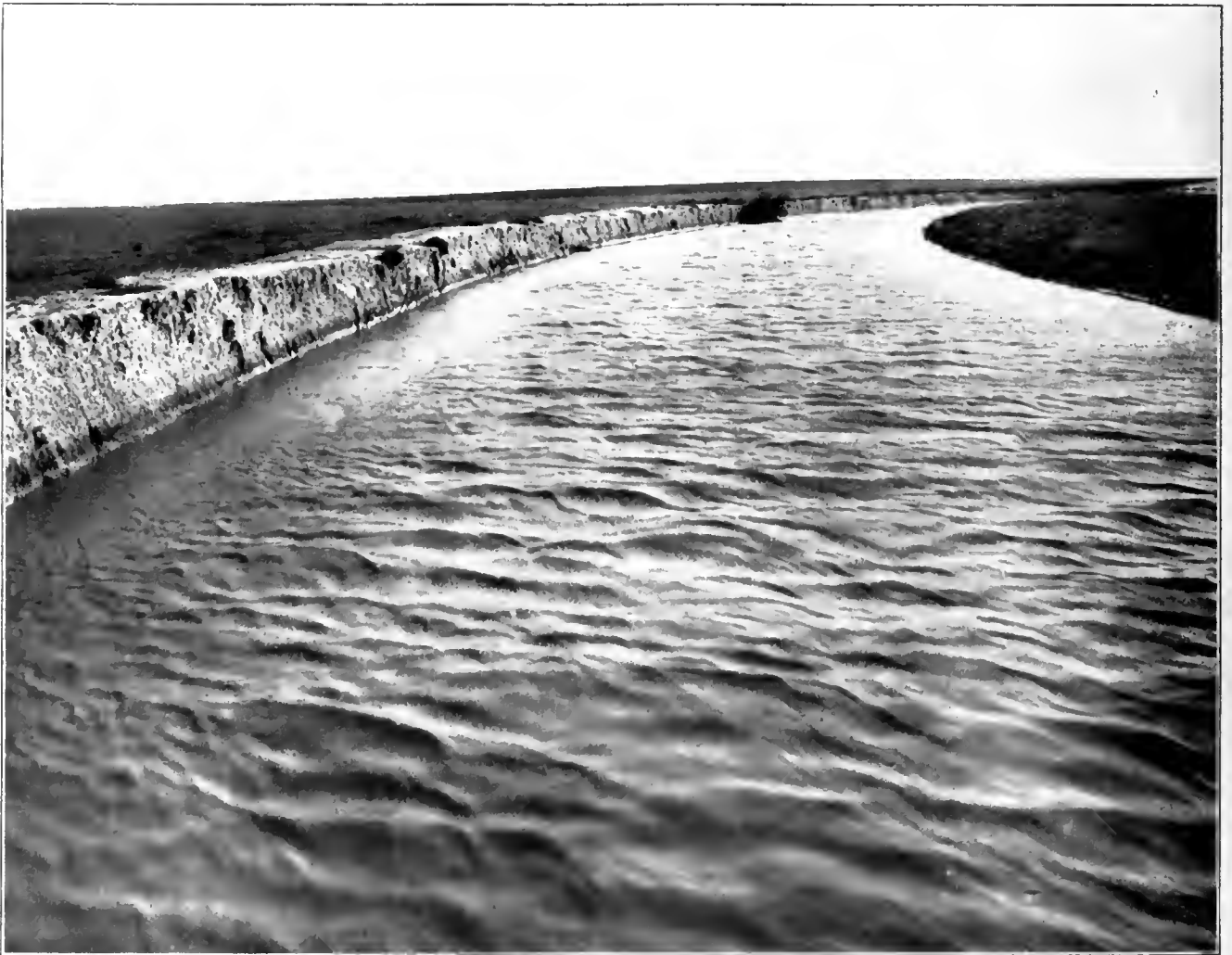
View on Kicking Bird Canal. This canal is the inlet to the reservoirs. It is 36½ miles long and although not full when this view was taken, it is 60 feet wide on the surface of water. It has a capacity of 1,000 second feet.
