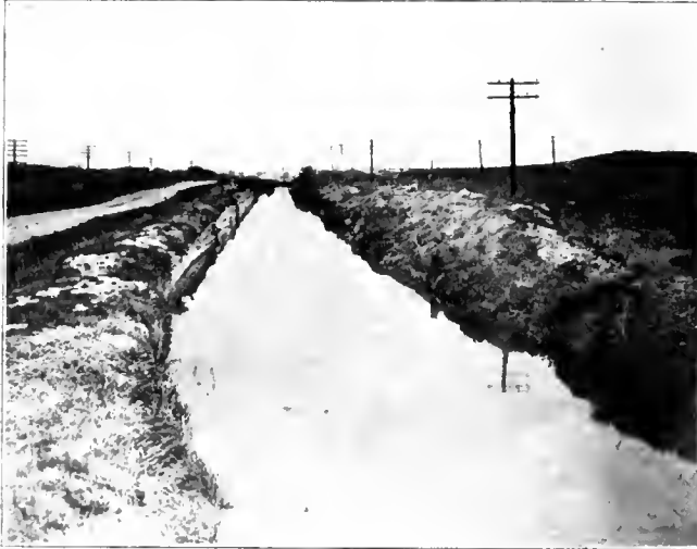
View of Main Canal of Fountain Valley Land & Irrigation Company's Project—2 Miles from Colorado Springs.
