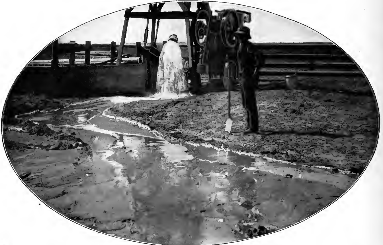
CENTRIFUGAL PUMP AND GASOLINE ENGINE IRRIGATION OUTFIT.
