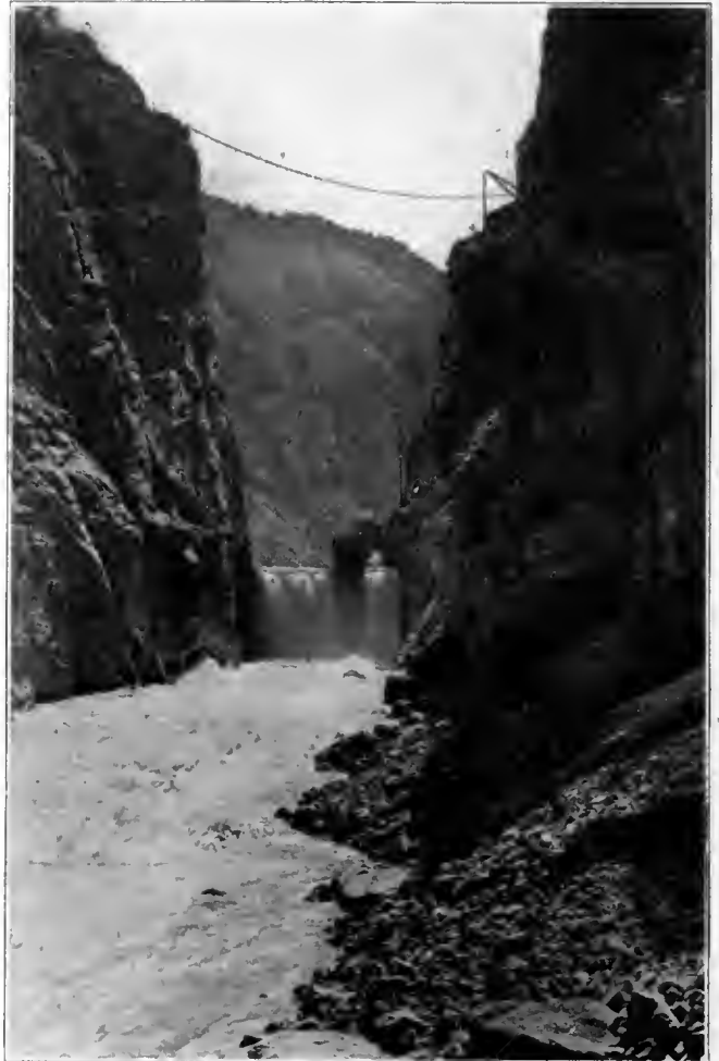
Shoshone Dam, General View of Dam Looking Up Stream, Shoshone Project, Wyoming.
