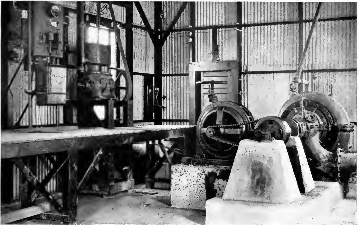
Interior Pumping Station No. 1, Patterson Ranch, California.
