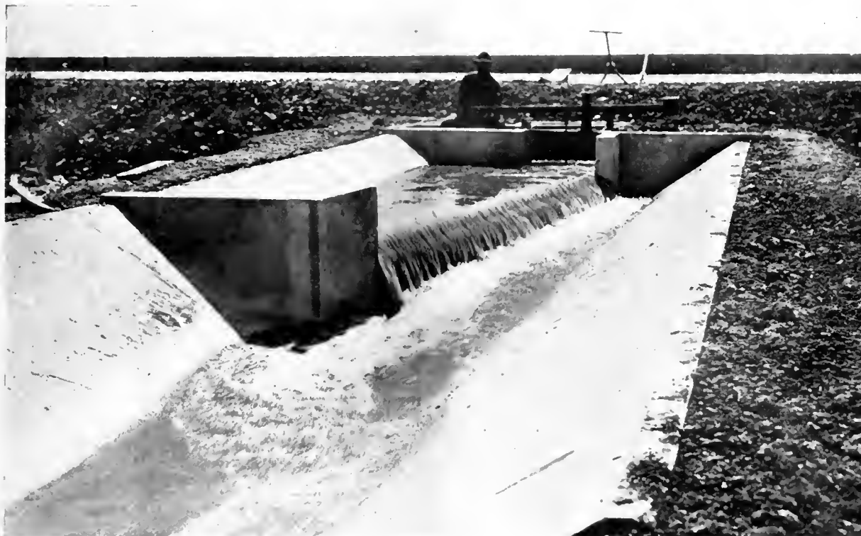
Showing Weir Conducting Water from Main Canal to Lateral, Patterson Ranch, California.
