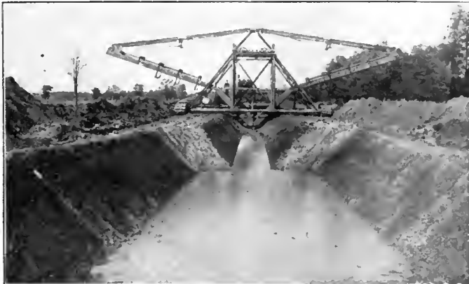
Ditch Being Dug with Sloping Banks—An Austin Drainage Excavator Ditch.
