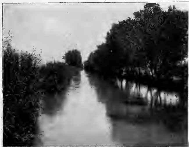
Main Canal, Mesa Project, Arizona.
