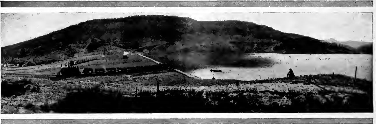
Schaeffer Dam, Under Construction, May 25th, 1910, Lake MacNeill, 35 Feet Deep, Will Be 90 Feet Deep When Completed.
