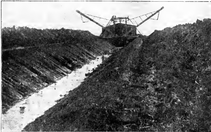
Ditch Being Dug by the Austin Drainage Excavator, 1½ to 1 Slope
