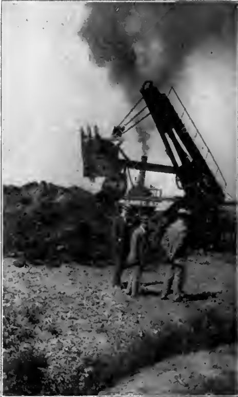
Constructing a Ditch, Showing Steam Shovel in Operation.
