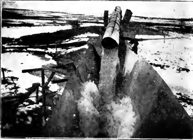
Water flowing from discharge pipe of pump. This flow, through a 10-inch discharge pipe, is 800 gallons per minute. This flow in summer, when cold will not retard it, is about 1,100 gallons per minute.
