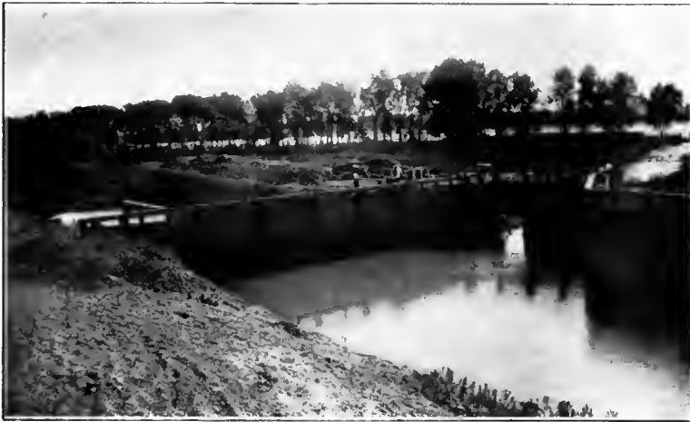
View at Spillway of Ditch—Cimarron, Kansas.
