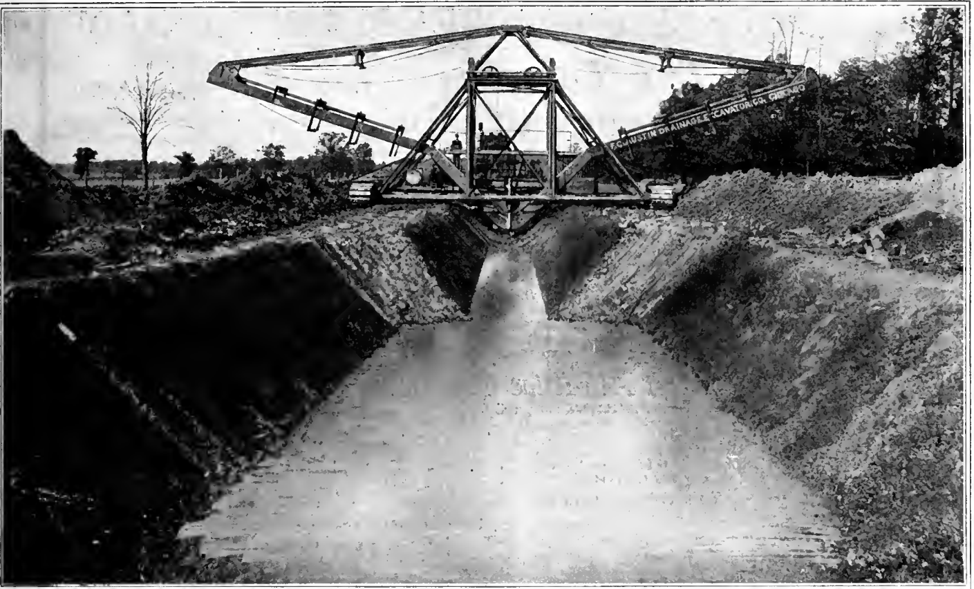
The illustration is a reproduction from a photograph of the Type "A" Austin Drainage Excavator mounted on rolling platform traction instead of track, each side of the machine having a bearing surface of 81 square feet, hence will travel over soft ground without much trouble. The cut also shows the different sized ditches that the machine is capable of digging. The first cut is an 18-foot bottom. The upper ditch is 4-foot bottom, about 8 feet deep and 1 to 1 slopes.
