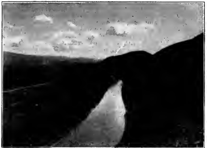
Shell Creek Canal in Big Horn County on Which Construction Has Recently Been Finished.
