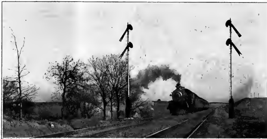
Automatic block signals on double track, between Seymour and Sarpy, on the Summit Lane Cut-Off.
