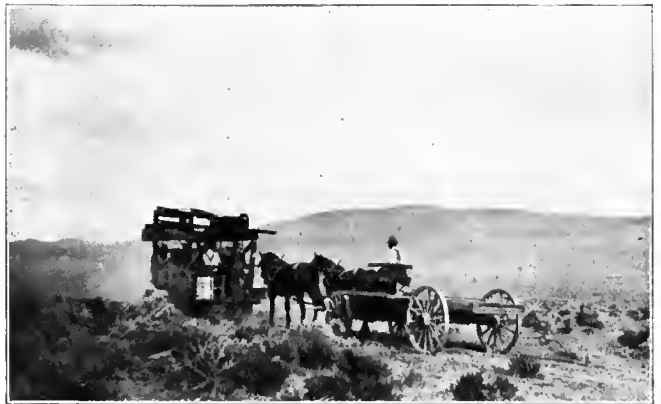
No. 3. Traction Gasoline Machine crossing the high Sierras of Eastern Washington, where fuel and water are not to be had. We made the 25 mile move in 8 hours, using 20 gallons of gasoline at 19c per gal. We had no team nor needed any. The one in the picture did not belong to the machine.
