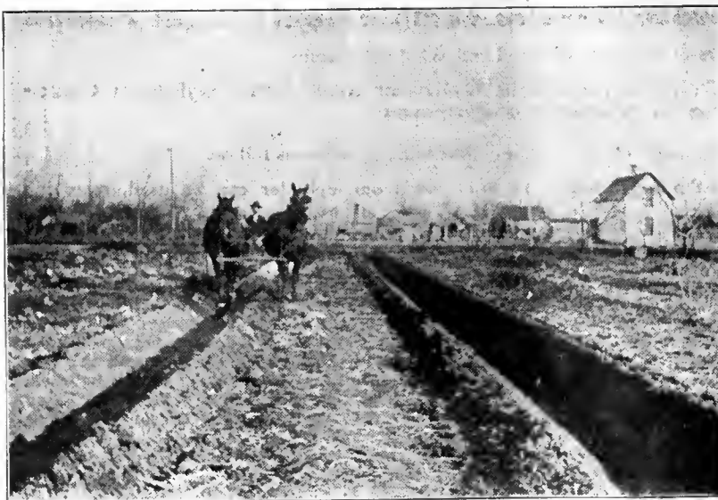
No. 1—20th CENTURY CUTTING "V" SHAPED LATERAL
