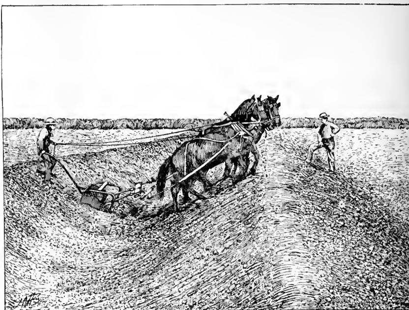
Fig. 21.—Building a supply ditch.
