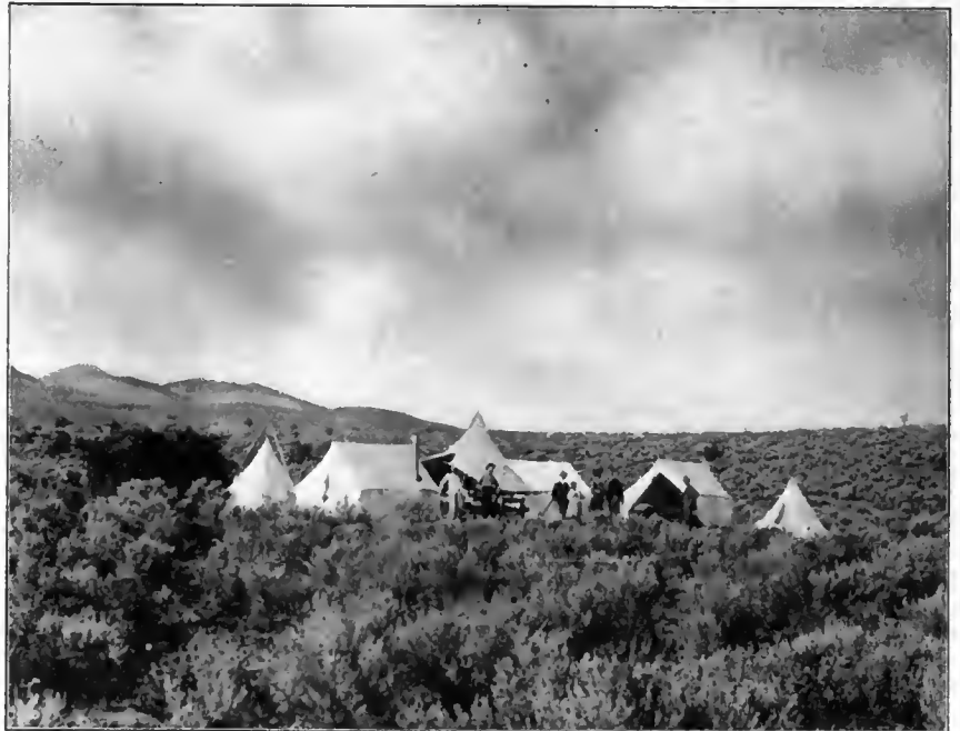
Engineers' Camp on Property of the Ranchos Orchard & Land Co.
