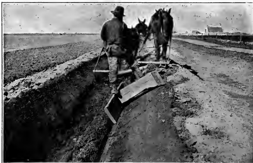
Fig. 8.—The Use of the "A" Scraper in Building Head Ditches.
