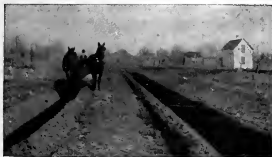
Cutting ditch 20 inches deep—24 inches wide.
