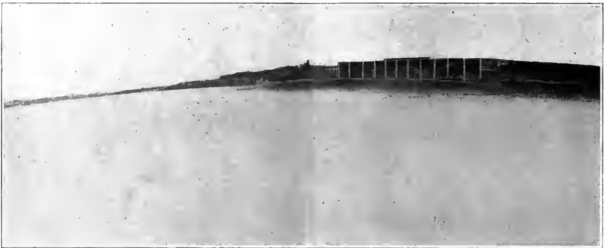
Headgates of the Arno Canal. At this point the canal taps the Pecos River and carries the water 15 miles to the waste-way, where the water is turned back to the river with a fall of 60 feet.
