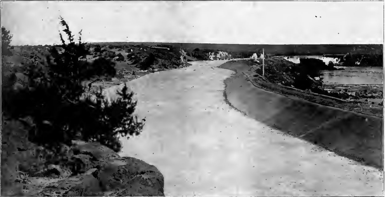
Main irrigation canal, Twin Falls North Side tract, showing new concrete lining. Width of canal at bottom, 65 feet. Perpendicular height of concrete walls, 9 feet. Milner dam in distance.
