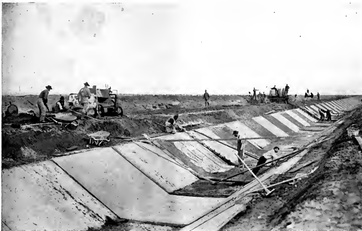
Cement Construction Work on Main Canal, Patterson Ranch, California.
