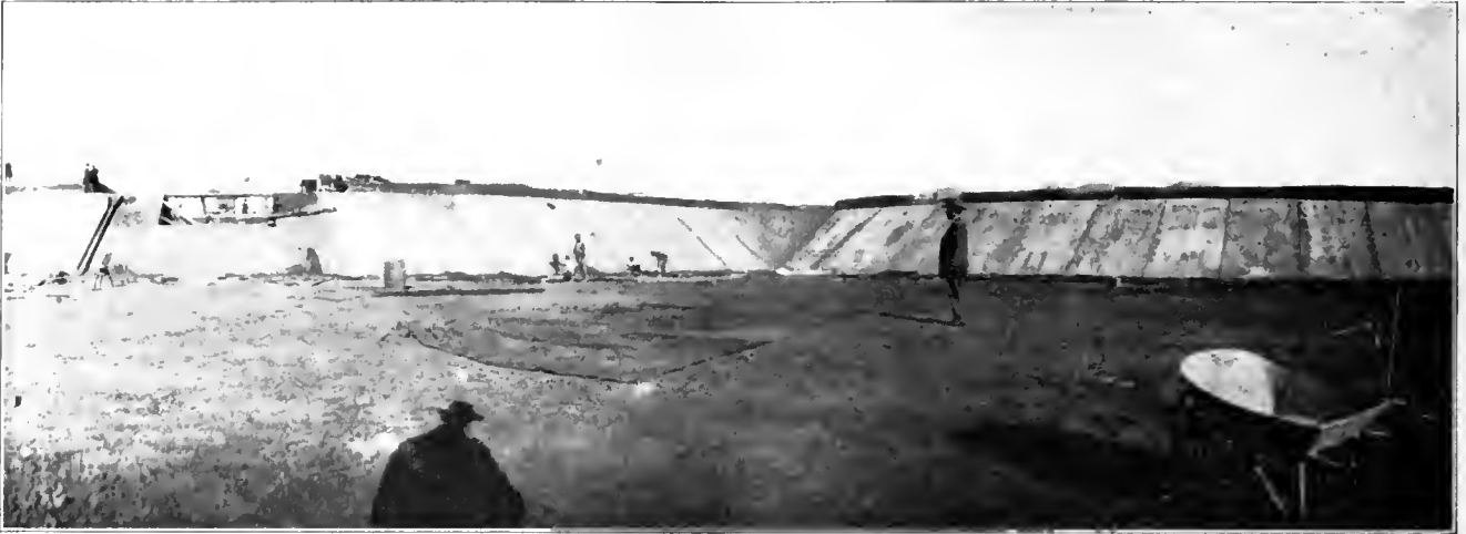
Constructing Cement Reservoirs, Patterson Ranch, California.
