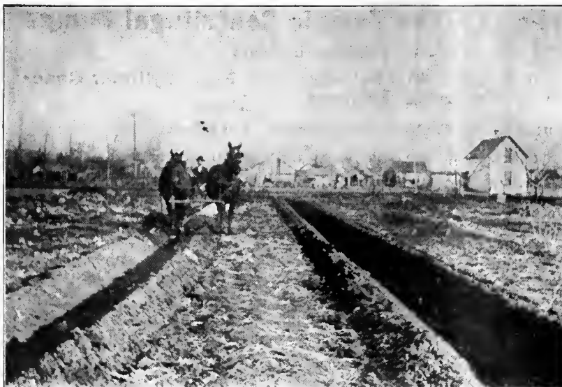
No. 1—20th CENTURY CUTTING "V" SHAPED LATERAL
