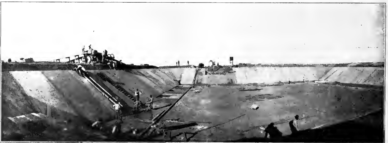
Construction Work on Cement Reservoirs, Patterson Ranch, California.
