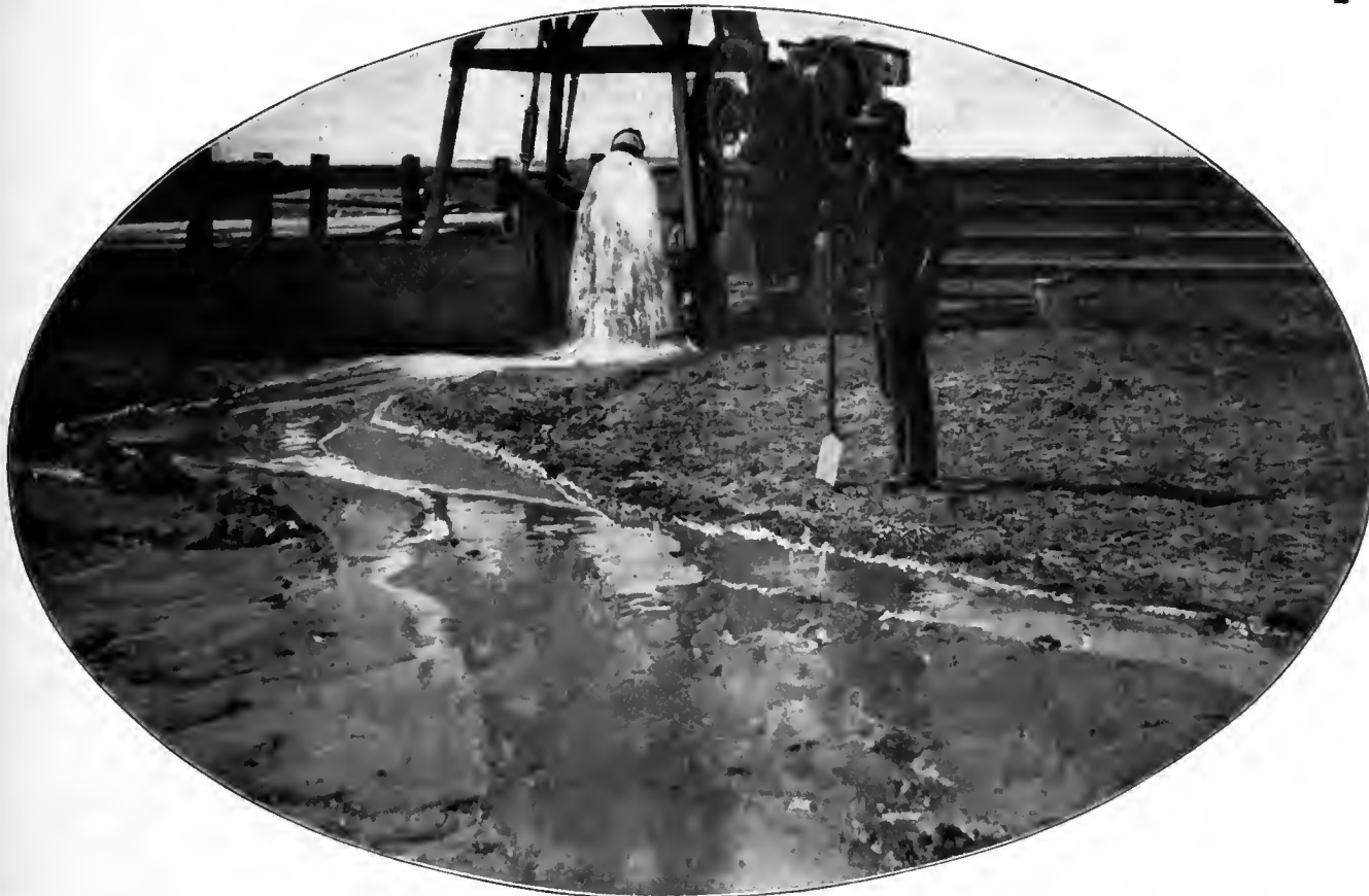
CENTRIFUGAL PUMP AND GASOLINE ENGINE IRRIGATION OUTFIT.
