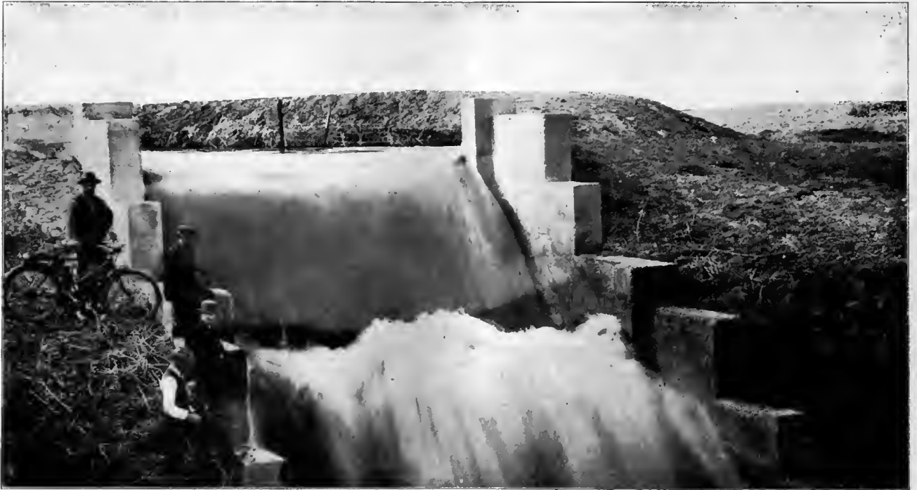
One of the Eleven Drops in the Comanche Canal, Arkansas Valley.
