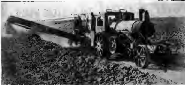
An Avery Undermounted Traction Locomotive pulling an Excavating Grader
