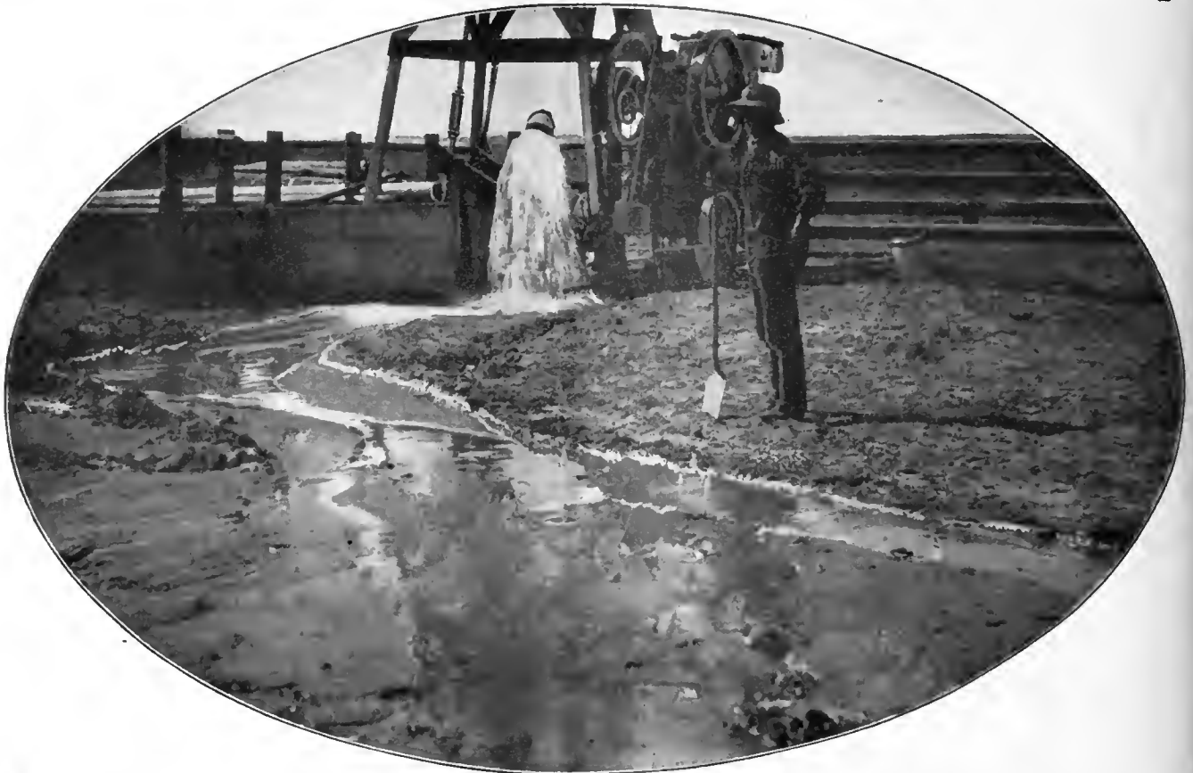
CENTRIFUGAL PUMP AND GASOLINE ENGINE IRRIGATION OUTFIT.
