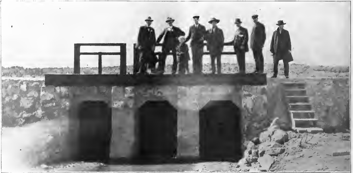
Type of small Diversion Dam and Waste Gate used in improving coulees in the Twin Falls North Side Irrigation System and concrete work used throughout this extensive system.
