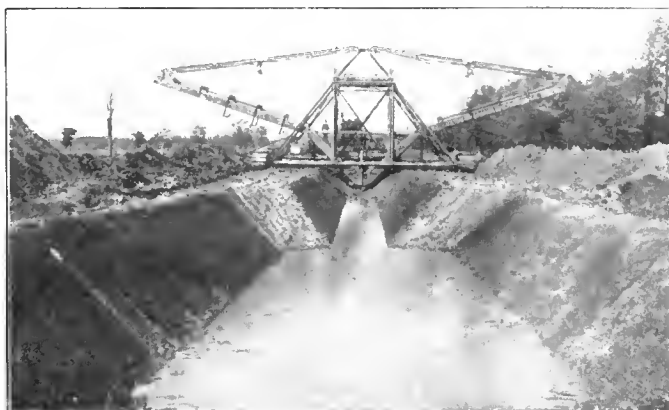
Ditch Being Dug with Sloping Banks—An Austin Drainage Excavator Ditch, showing variations in width made by same machine
