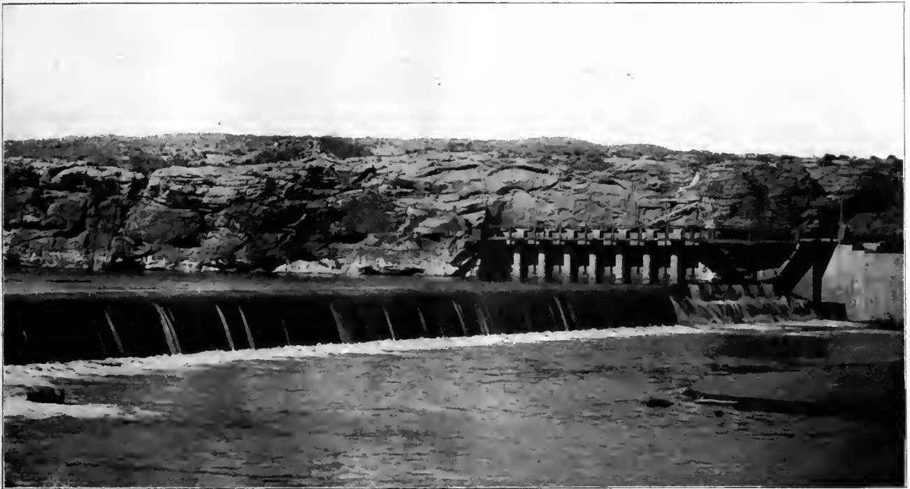
Dam in the Arkansas River. Arkansas Valley Sugar Beet & Irrigated Land Company's Project.
