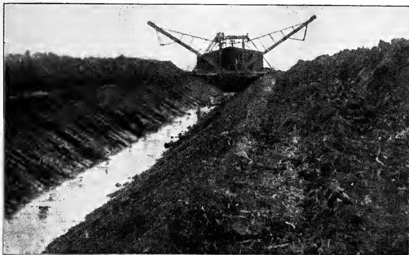
Ditch being Dug by the Austin Drainage Excavator, 1\frac{1}{2} to 1 Slope
