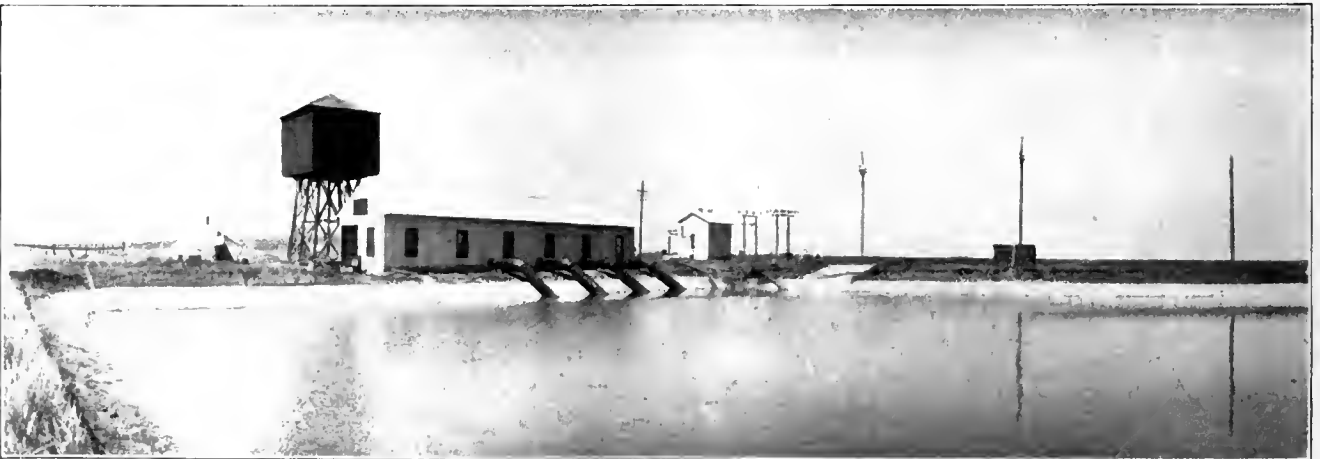
Showing Transforming Station of Power Line, Which Furnishes Electric Power for Patterson Irrigation System, Situated at Reservoir No. 1.
