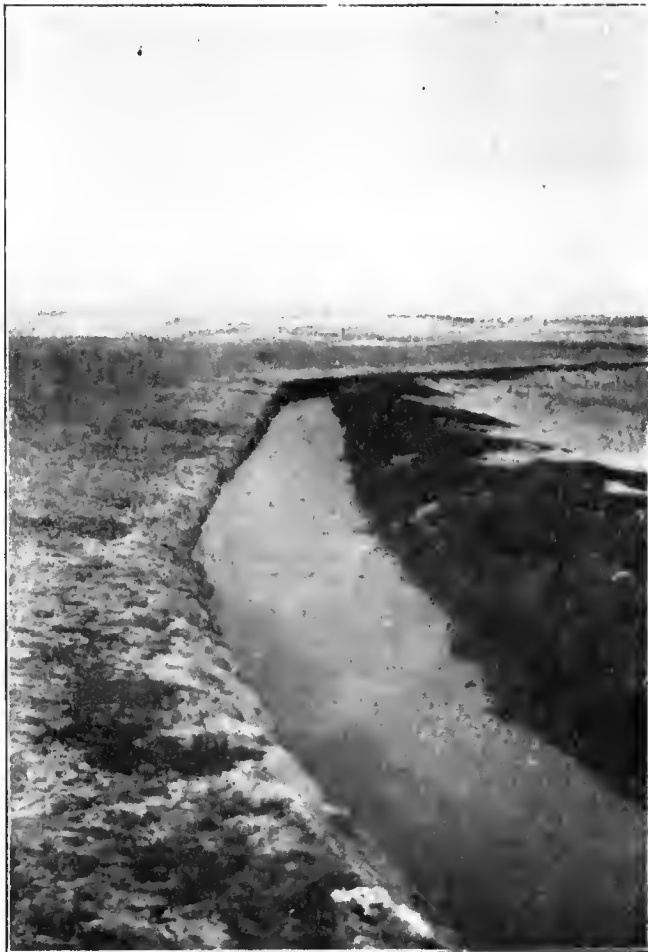
View of ditch about 1,000 feet from pumping plant.
