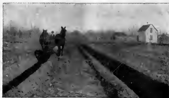
Cutting ditch 20 inches deep, 24 inches wide
