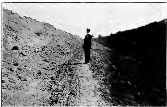
View of Main Canal, Nearly Completed.
