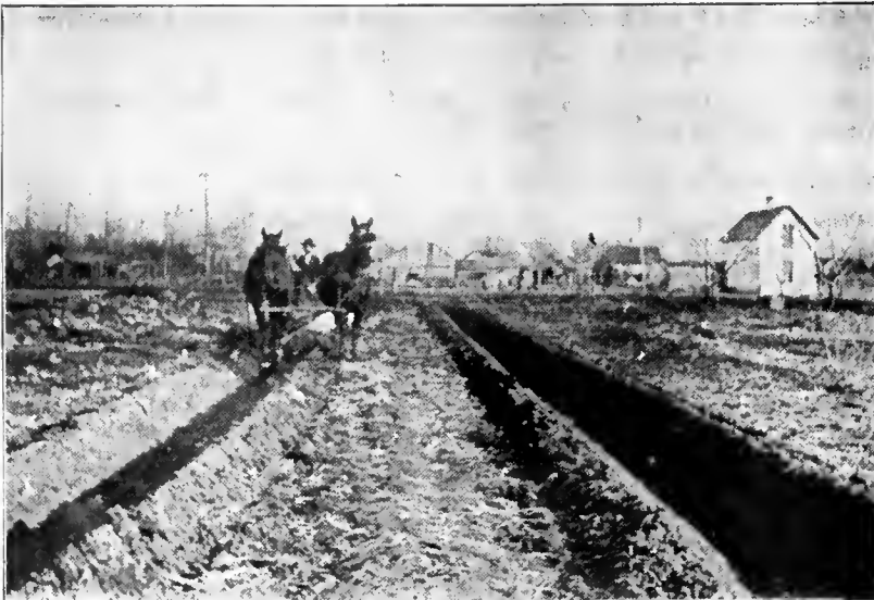
No. 1—20th CENTURY CUTTING "V" SHAPED LATERAL
