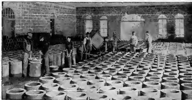
Making Cement Pipe for Irrigation and Sewers
