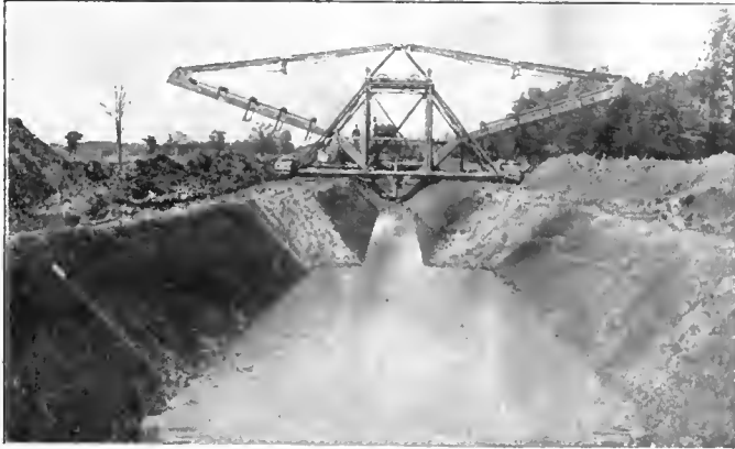
Ditch Being Dug with Sloping Banks—An Austin Drainage Excavator Ditch, showing variations in width made by same machine
