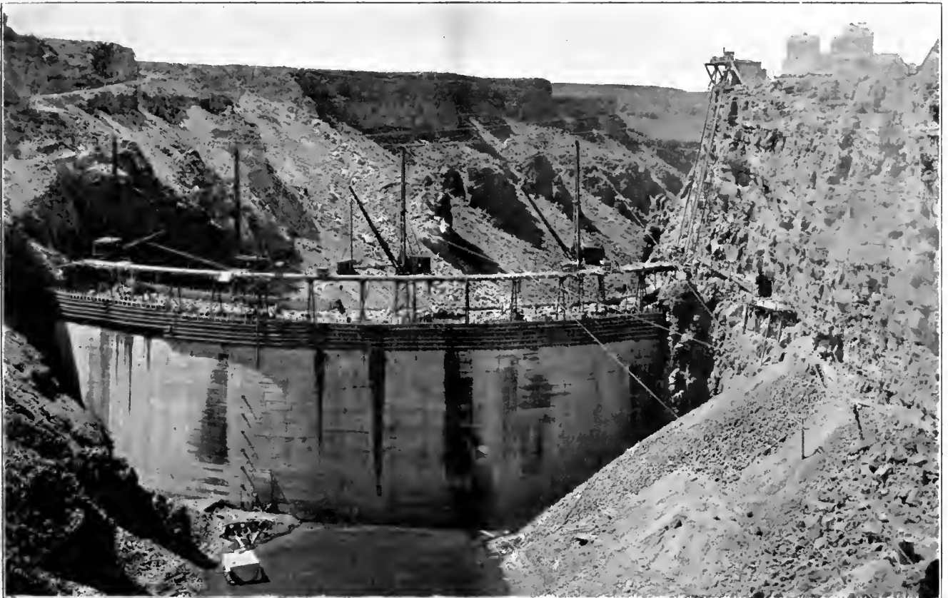
Down Stream View, July, 1910.—Salmon River Dam.
