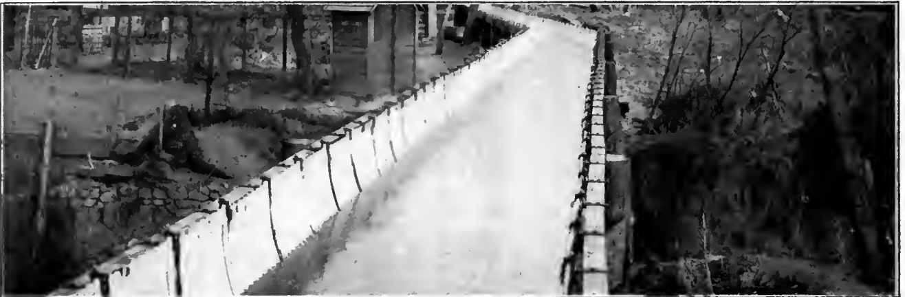
One of Our No. 93 Flumes Erected for the Stratton Estate, Colorado Springs. Capacity 40 Cubic Feet Water per Second on a Grade of Five Feet to the Mile.
