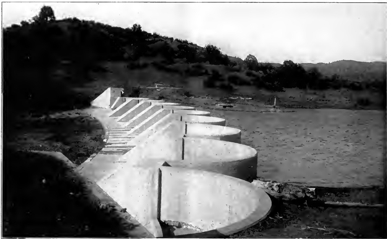
SPILLWAY, ORLAND PROJECT, CALIFORNIA.
