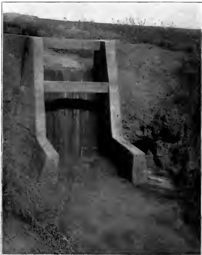
View Showing Concrete Construction on Canal Work Near Holly, Colo.
