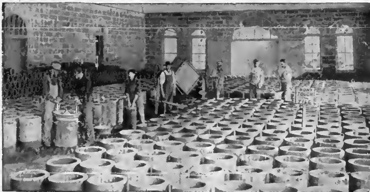
Making Cement Pipe for Irrigation and Sewers
