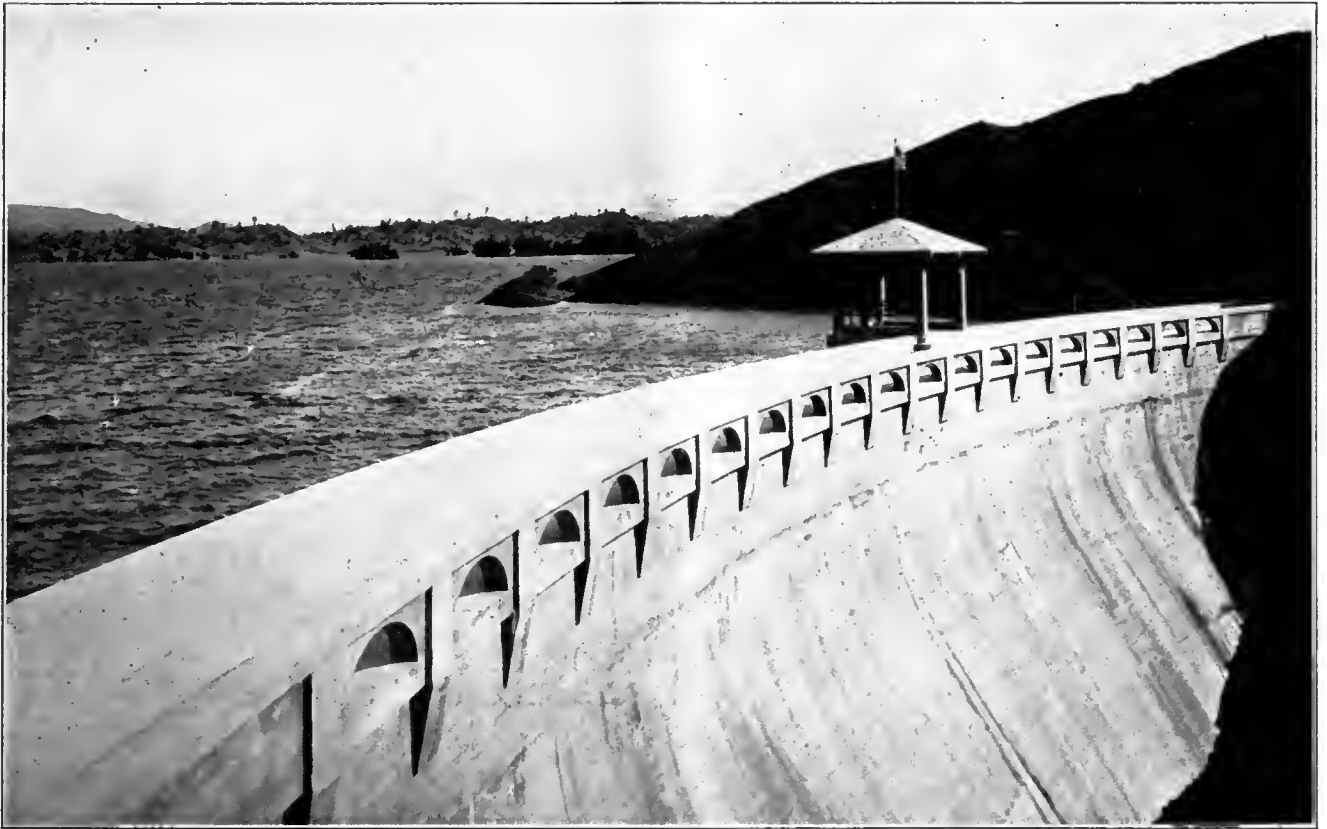
DAM AT EAST PARK, COLO., IMPOUNDING WATER OF STONY CREEK FOR USE ON THE ORLAND PROJECT.
