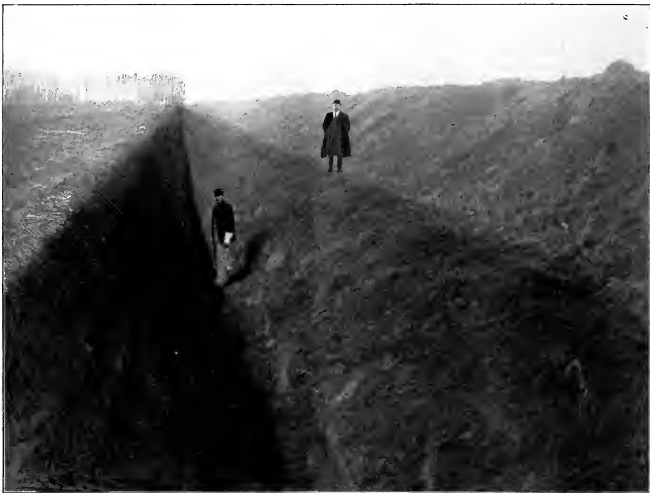
This shows a ditch dug by the Avery Traction Steam Shovel. It is claimed for the outfit which performed this work that it is more than a steam shovel, in other words it is a traction engine combined with the shovel. The same engine may be used by a rancher on a combined cultivator, for hauling, plowing, belt-work, traction work, grading, driving stone crusher and pulling road grader. This engine is made by the Avery Company, Peoria, Ill.
