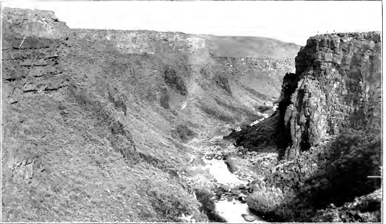
Canon Before Any Work Was Done.—Salmon River Dam.
