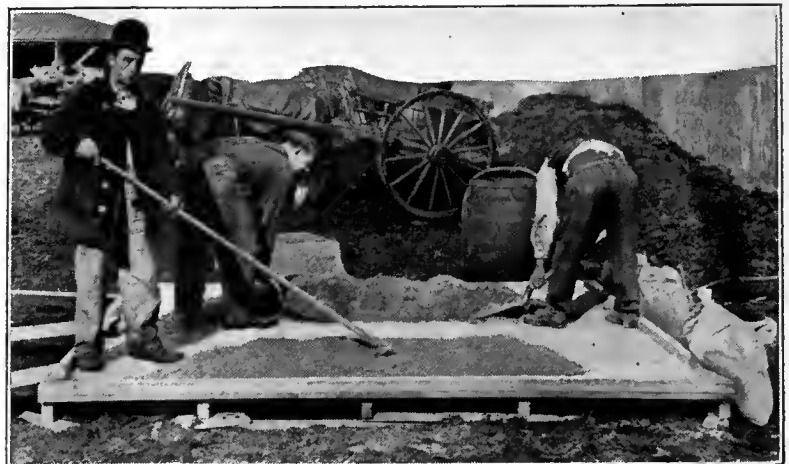
Men Shoveling and Man Raking Concrete.
