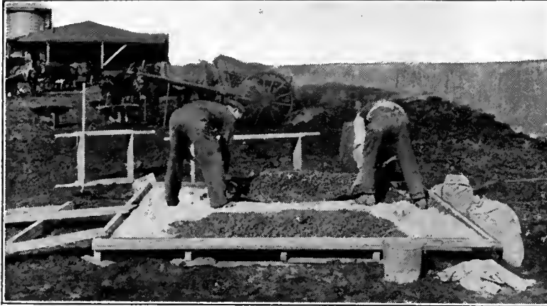
Men Shoveling Concrete.
