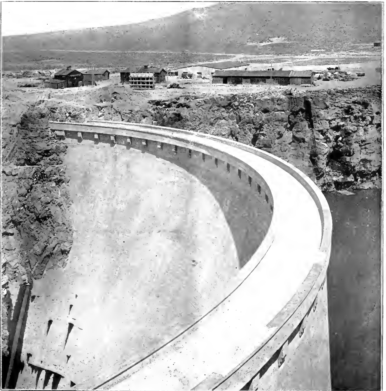
View from Cliff at West End, Looking Down on Top. Salmon River Dam, May, 1911.
