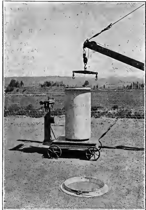
Fig. 27.—Tank Experiments at Reno, Nev., to Determine Effects of Soil Mulches in Checking Evaporation.
