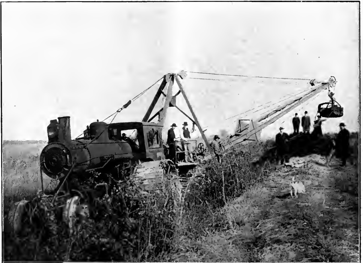
Avery Steam Shovel owned by Handy & Spangler, St. Charles, Mo., at work on their farm, building a levee. This outfit is manufactured by the Avery Company, Peoria, Ill., and is used also for irrigation work, drainage, street excavating, stripping coal, etc. In the April issue of this journal will be shown a fine ditch opened out by this outfit.
