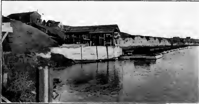
GENERAL VIEW SHOWING PUMPING STATION.
