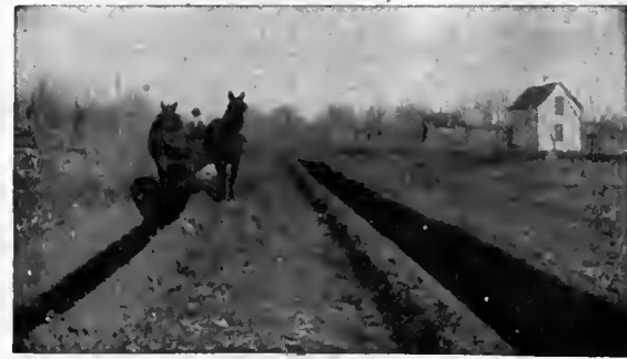
Cutting ditch 20 inches deep, 24 inches wide
