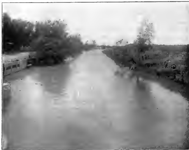
View of Main Canal Near Holly, Colo.
