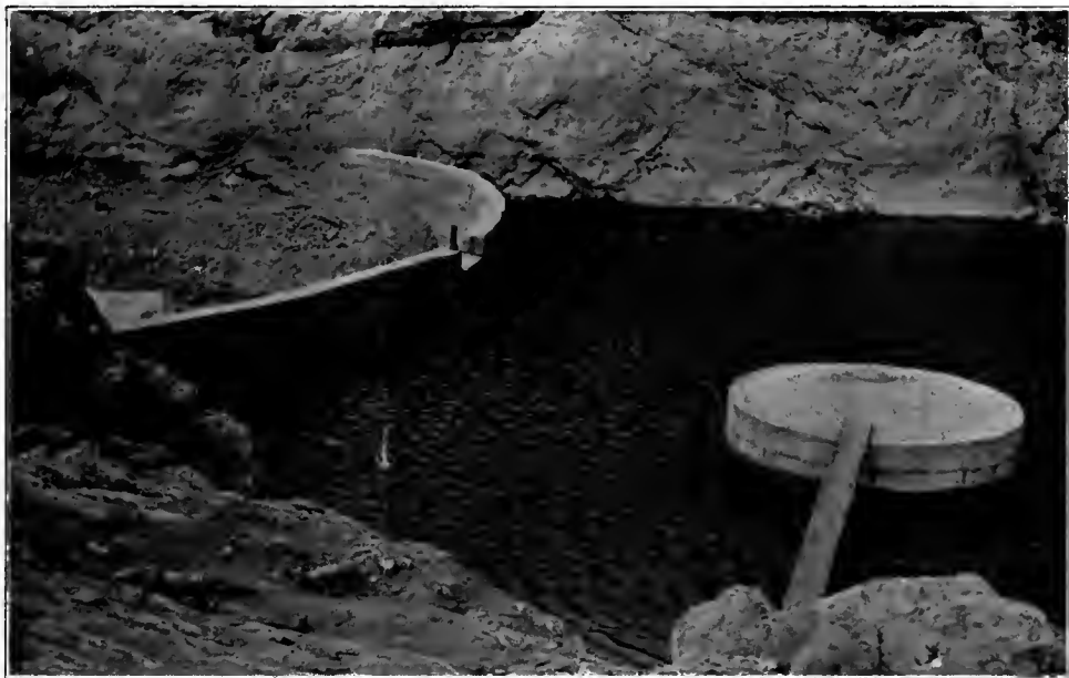
Fig. 2. View of Sub-Surface Dam and Collecting Head.
