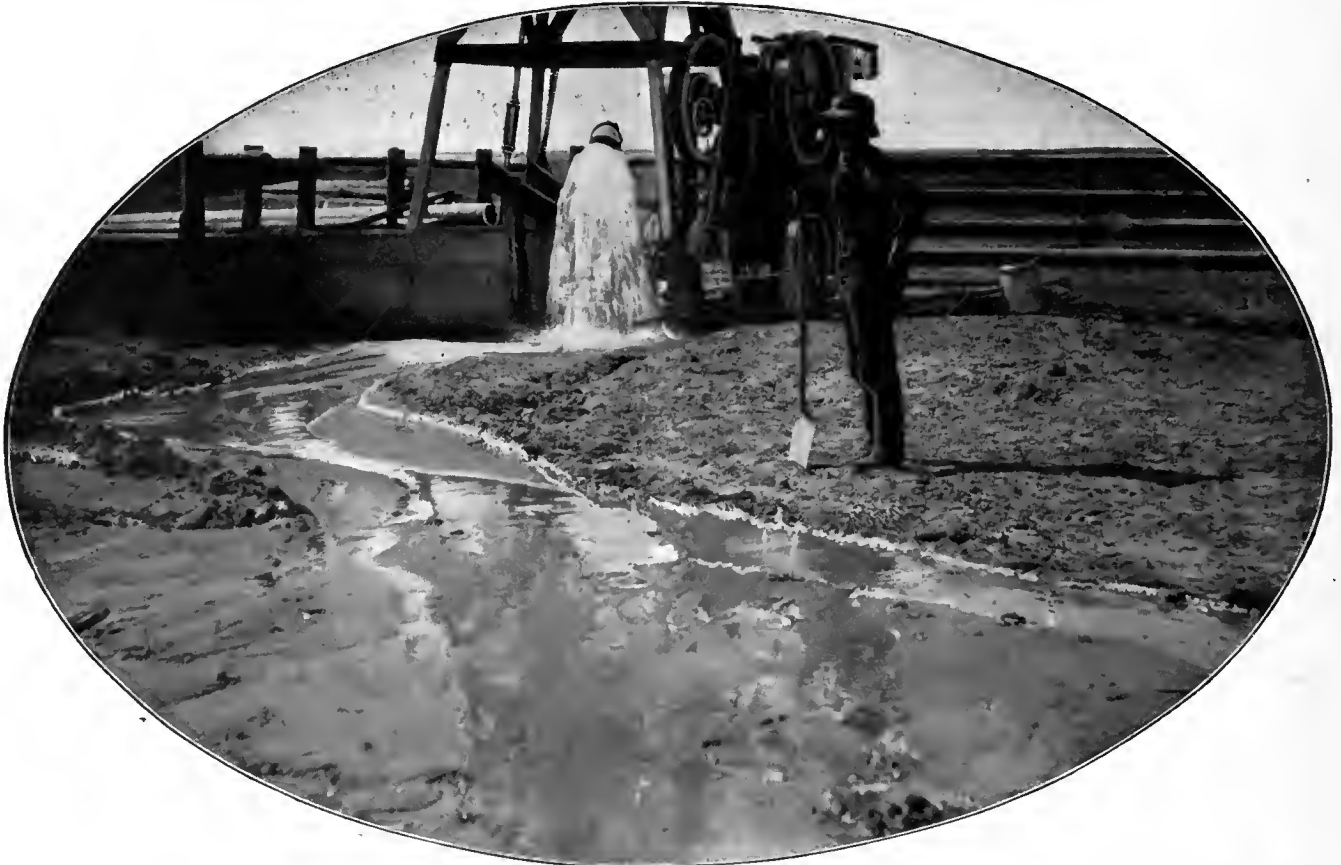
CENTRIFUGAL PUMP AND GASOLINE ENGINE IRRIGATION OUTFIT
