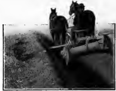
Cutting V-Bottom ditch on Slope of 1\frac{1}{2} to 1.
