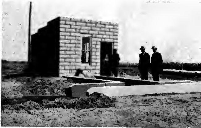
The irrigation pump house on the poor farm at McCook, Neb. The pump delivers an 8-inch stream against a 90-foot head.
