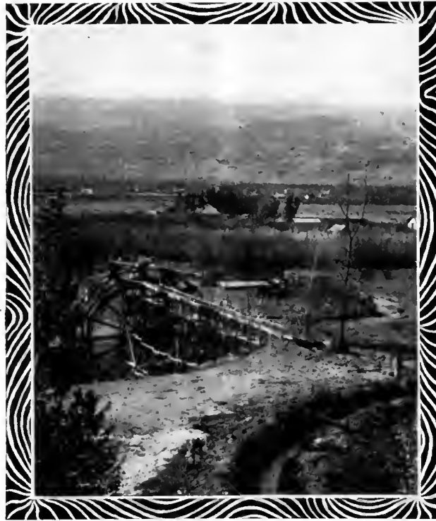
A water wheel which lifts irrigating waters from Grand River in Colorado.
