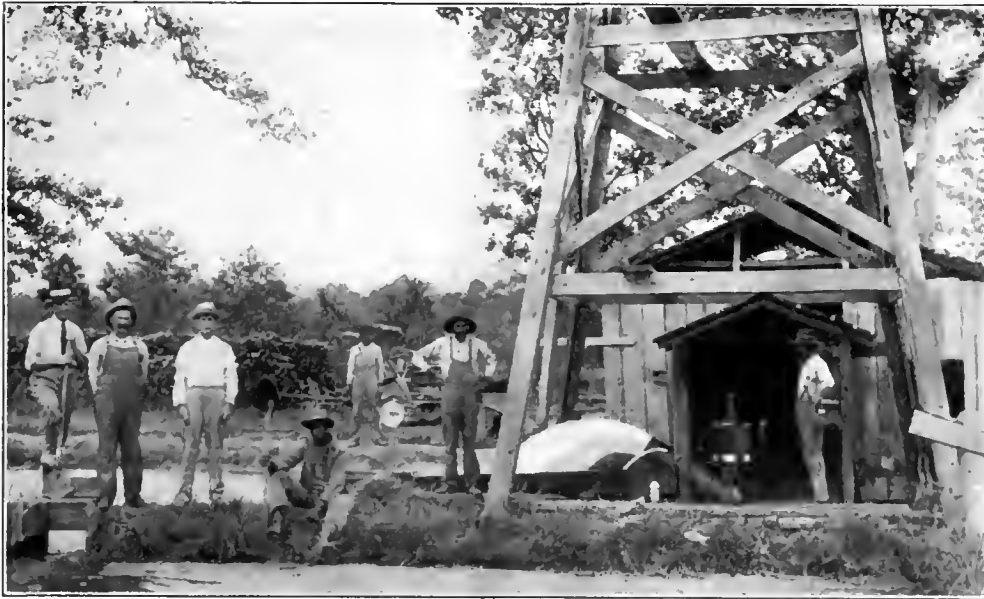
An Arkansas Installation. Layne Patent Screen and Patent Enclosed Line Shaft Centrifugal Pump.
