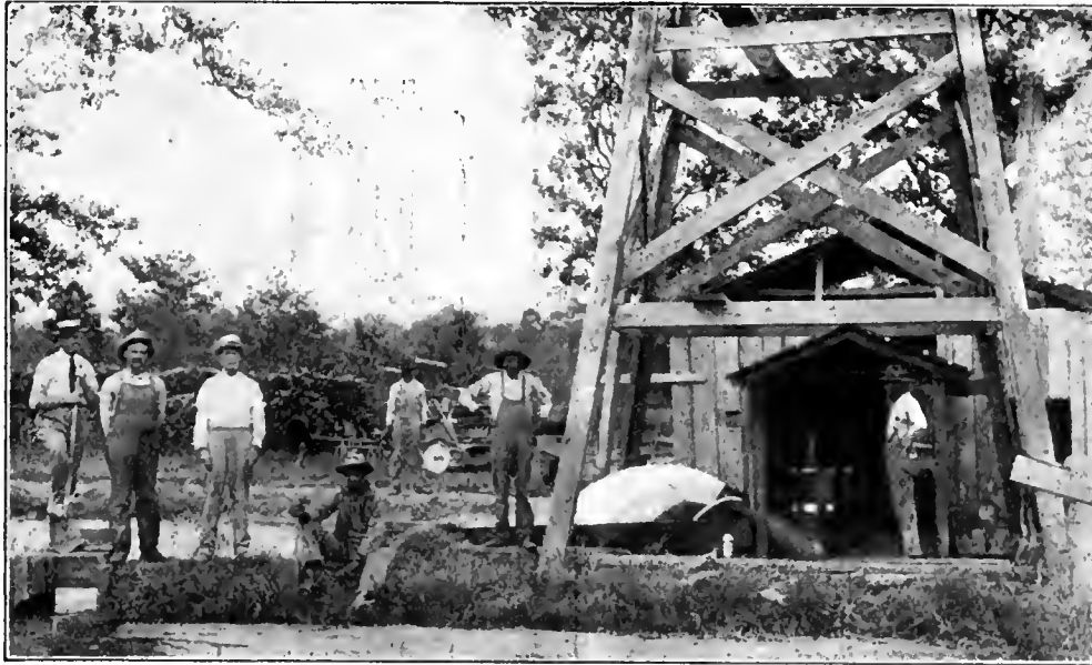
An Arkansas Installation. Layne Patent Screen, and Patent Enclosed Line Shaft Centrifugal Pump.
