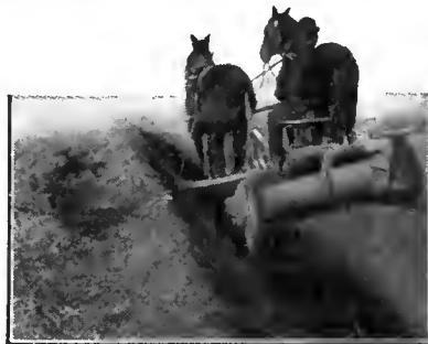
Cutting V-Bottom ditch on Slope of 1\frac{1}{2} to 1.
