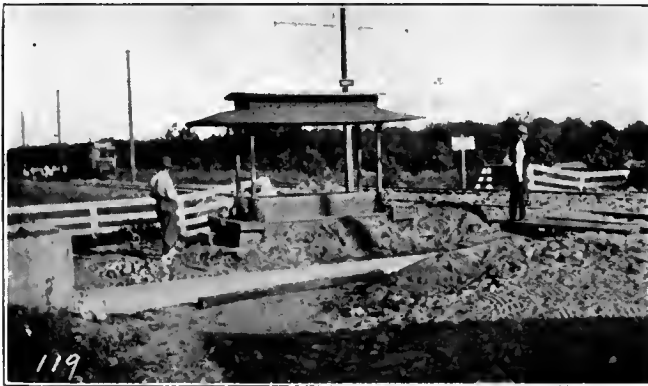
Installing Pure Iron Culvert Under Tracks of Interurban Railway.
