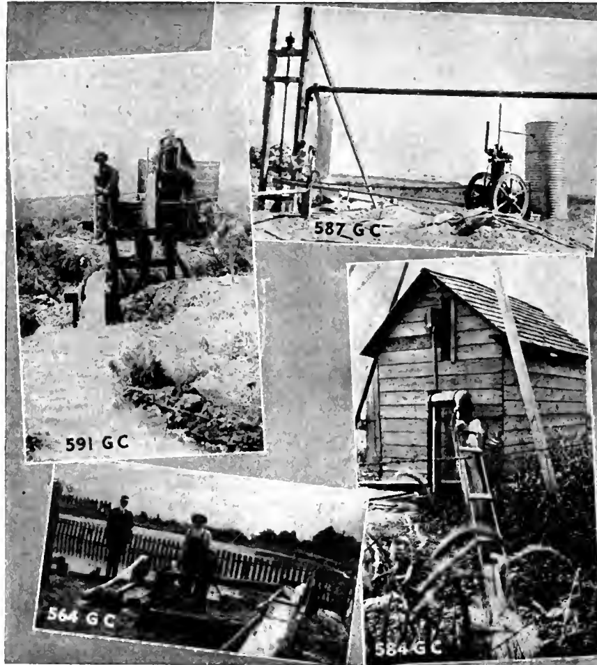
Small irrigation plants in Idaho and Utah—587GC is a pumping plant made up of a 9 H. P. Vertical Oil Engine and 3-inch Vertical Centrifugal Pump. This pump is in a 60-foot pit. Plant at Lehi, Utah. 591GC is a plant located at Springfield, Idaho. This consists of a 3-inch Vertical Centrifugal Pump being driven by a 2 H. P. engine, delivering 350 gallons per minute into the irrigation ditch. The engine is mounted on a farm wagon and can easily be moved to other wells or used for other power purposes. 584GC is located near Bountiful, Utah, and consists of a 4 H. P. engine with walking beam operating a 6-inch cylinder at a depth of 72 feet. 564GC is located at Layton, Utah, and consists of a 5 H. P. Motor driving a 5-inch Centrifugal Pump which delivers about 800 gallons per minute into the flume.—Courtesy of Fairbanks-Morse & Co.
