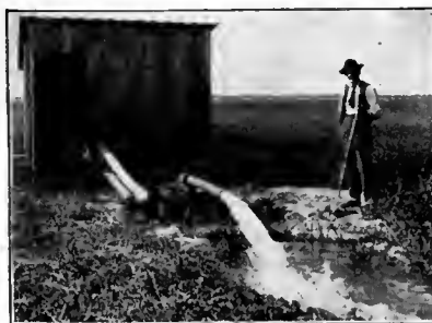
Irrigating Alfalfa with an 8 H.P. Fairbanks-Morse Oil Engine and Centrifugal Pump
