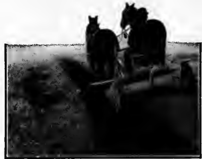
Cutting V-Bottom ditch on Slope of 1½ to 1.
