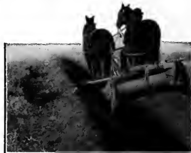
Cutting V-Bottom ditch on Slope of 1½ to 1.
