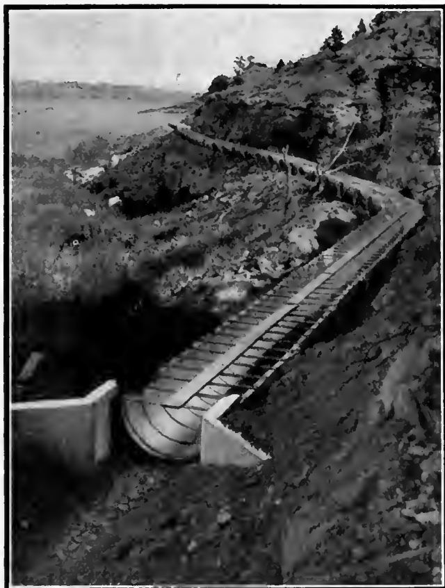
SECTION OF NEWCOMB FLUME ON UNITED STATES GOVERNMENT RECLAMATION PROJECT NEAR HUNTLEY MONT.
