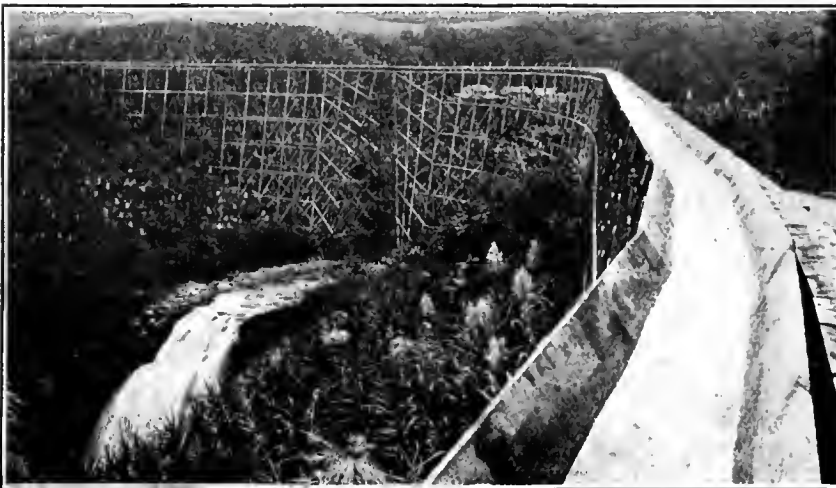
Cane Flume and Trestle Across Kawainui River near Pepeekeo, Hawaii.
