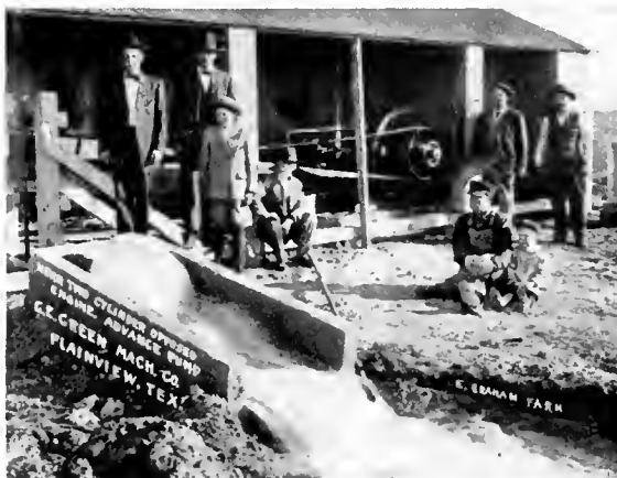
A Texas Pumping Plant
