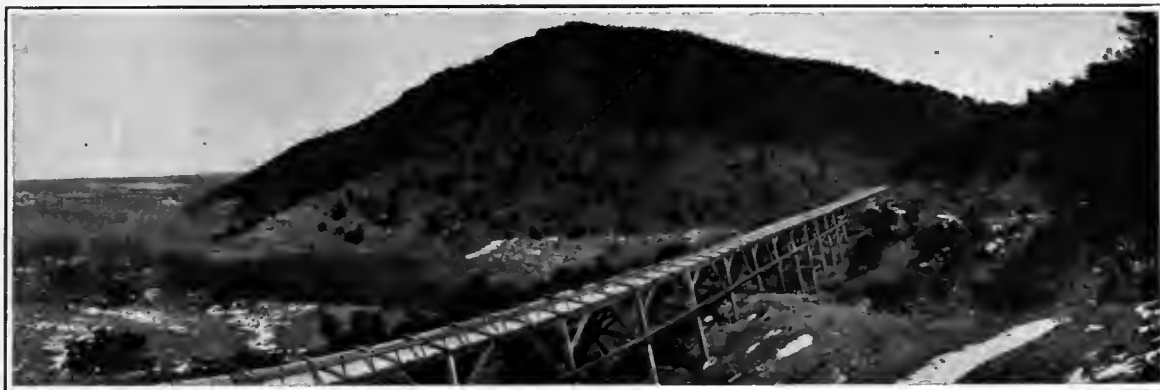
An Unusually Fine Section of Flume Work Erected by the Lennon Metal Flume Co., Colorado Springs, Colo.
