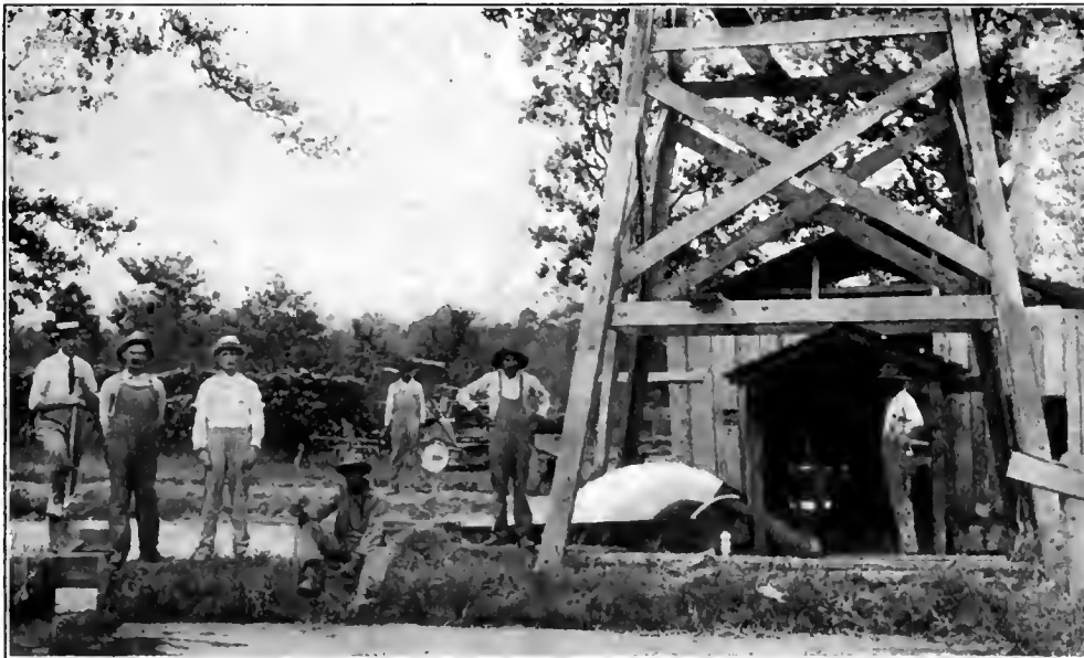
An Arkansas Installation. Layne Patent Screen and Patent Enclosed Line Shaft Centrifugal Pump.
