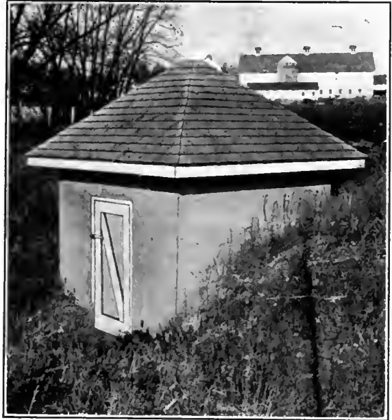
A Concrete Hydraulic Ram House on the Property of John F. Jelke, Dundee, Ill.
