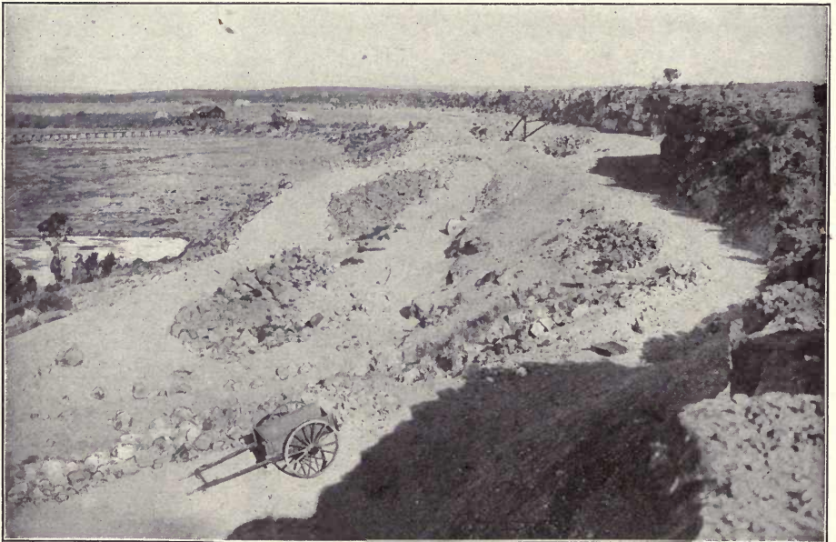
Construction work on Twin Falls North Side Canal.
