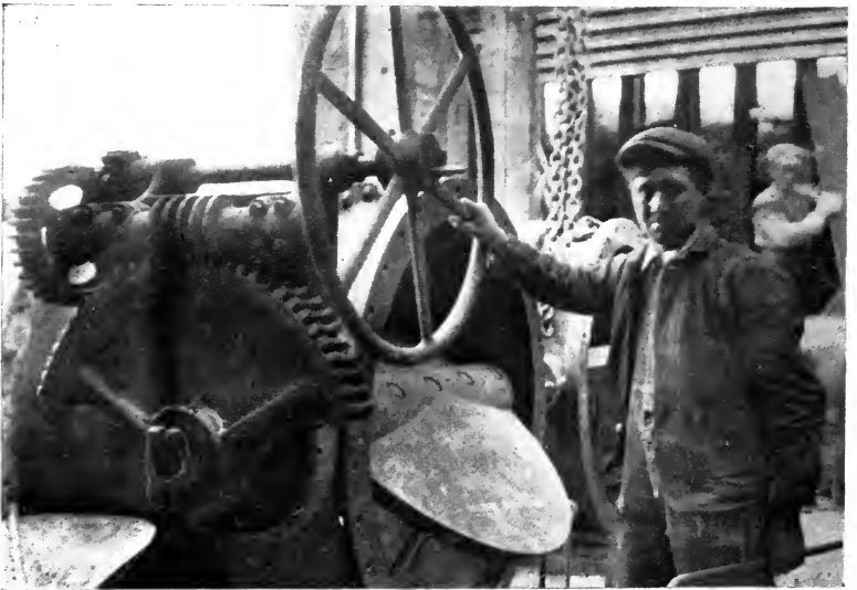
FIG. 174.—Butterfly Valve, Minitare Dam, Nebraska.
