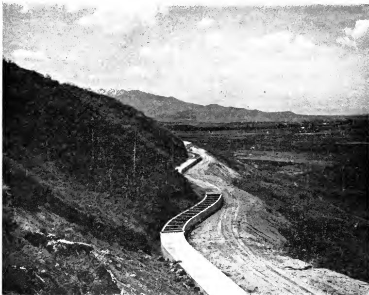
FIG. 162.—High Line Canal, Spanish Fork Valley, Utah, Covered to Protect against Land and Snow Slides.
