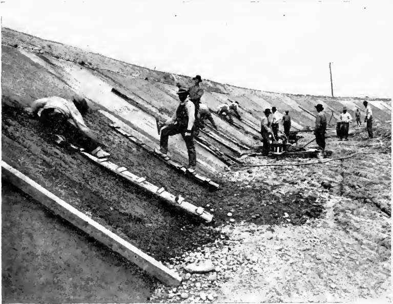
FIG. 84.—Lining Canal with Concrete, Idaho.
