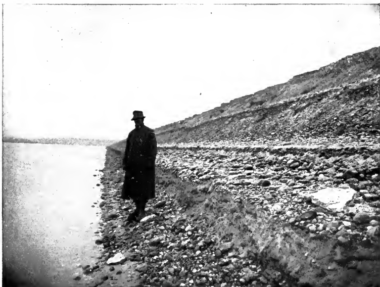
FIG. 202.—Upper Deer Flat Embankment, Showing Beaching of Gravel slope.
