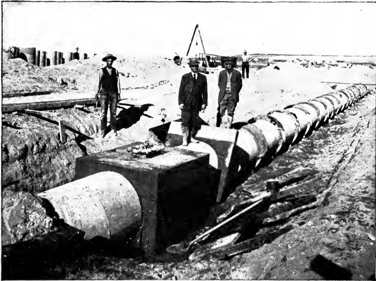
FIG. 161.—Manhole and Concrete Collars on Concrete Pressure Pipe. Boise Project.
