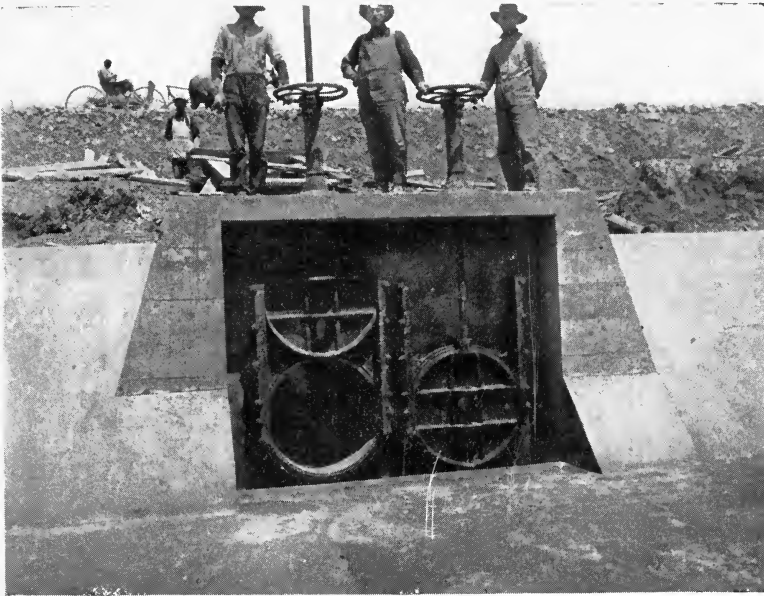
FIG. 105.—Cast-iron Valve on Small Lateral Turnout.
