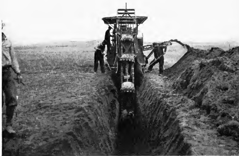
FIG. 61.—Excavating Trench for Tile Drain, Montana.
