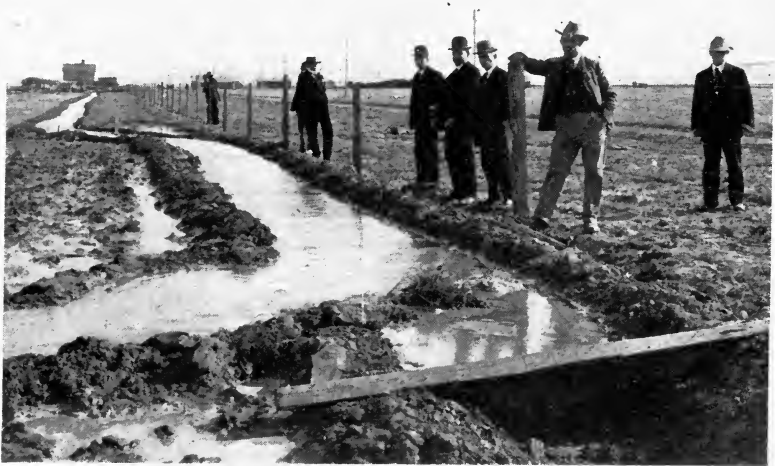
FIG. 33.—Diverting Water from Head Ditch by Canvas Dam, Shoshone Valley, Wyoming.
