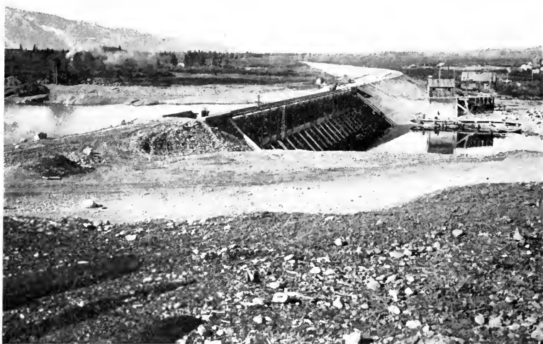
FIG. 98.—Jackson Lake Dam, Downstream Face, Wyoming.
