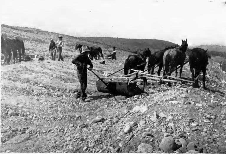
FIG. 77.—Building Canal with Fresno Scrapers.
