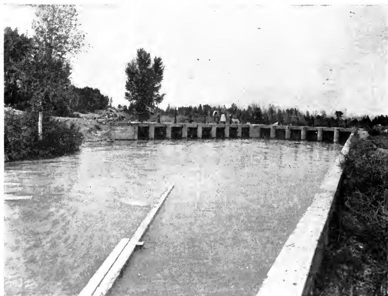
FIG. 99.—Headgates and Sluice Gates, Montrose and Delta Canal, Uncompahgre Valley, Colorado.
