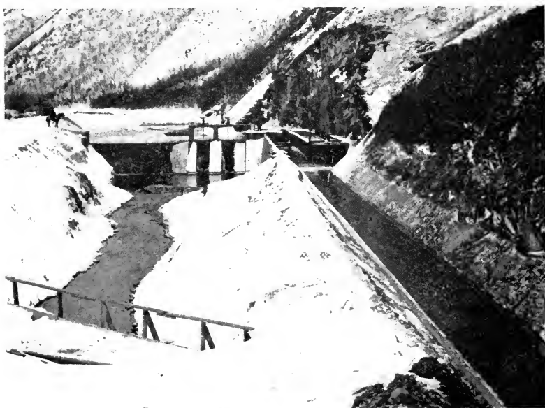
FIG. 163.—Headgates, Sluice Gates, and Sand Basins, High Line Canal, Spanish Fork Valley, Utah.
