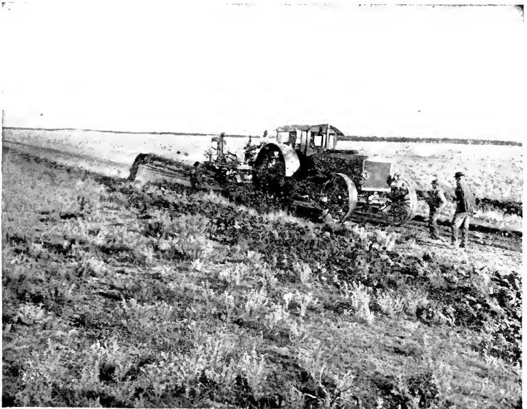
FIG. 75.—Building Lateral in Montana with Elevating Grader.
