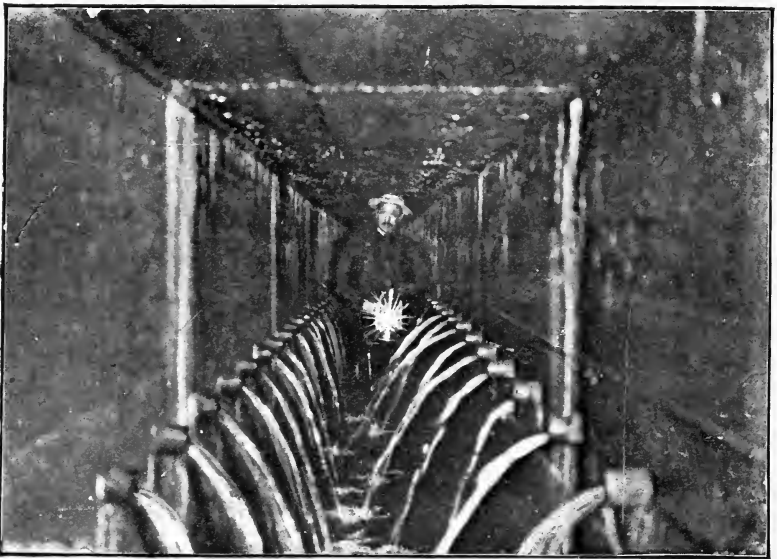
FIG. 14.—Subterranean Water Tunnel and Feed-wells: California.
