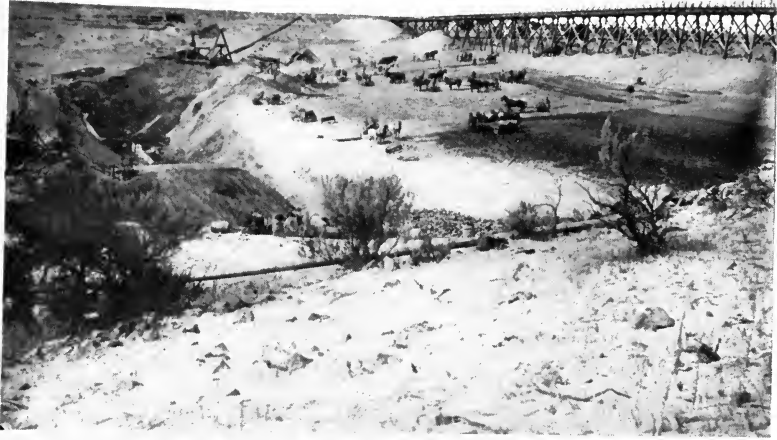
FIG. 204.—Cold Springs Dam under Construction, Umatilla Valley, Oregon.
