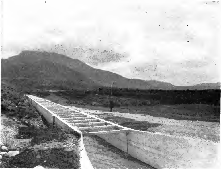
FIG. 146.—Concrete Flume, Spanish Fork Valley, Utah, showing Warped Transition from Canal to Flume.
