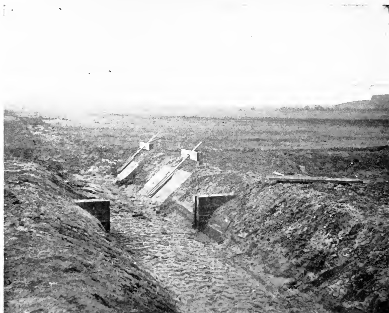
FIG. 104.—Check and Farm Turnout with Inclined Valve.
