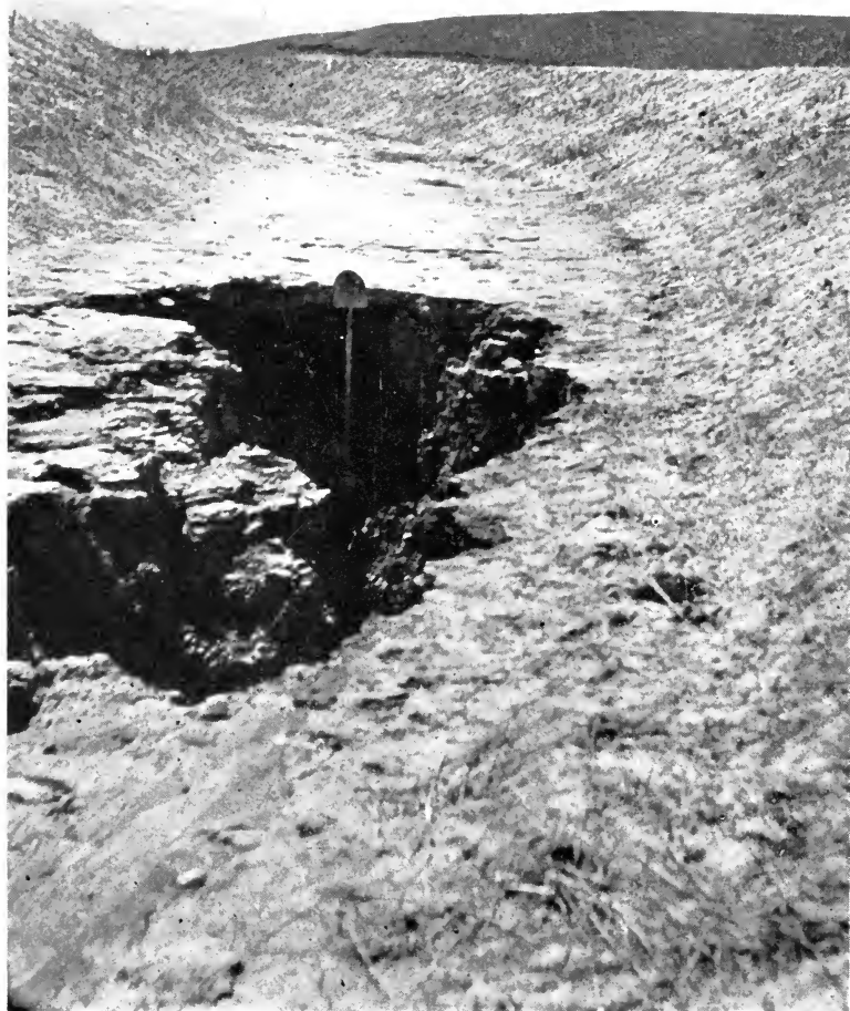
FIG. 73.—Cave Developed in Bottom of Canal, Flathead Indian Reservation.
