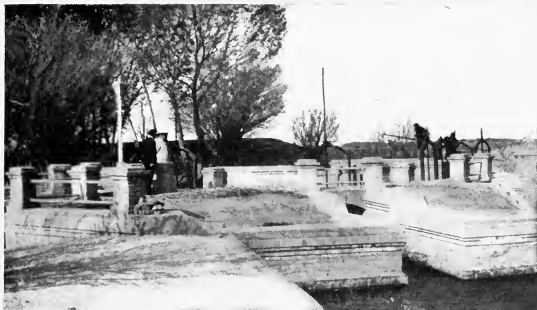
FIG. 100.—Division Gates and Drops on Tsar Canal near Byram Ali, Murgab Valley, Turkestan.
