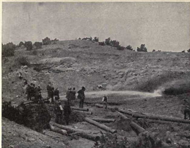
A. BUILDING DAM BY HYDRAULIC PROCESS AT SANTA FÉ, NEW MEXICO, SHOWING HYDRAULIC GIANT IN USE.
