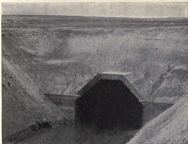
B. TUNNEL IN EARTH ON CROCKER-HUFFMAN CANAL, CALIFORNIA.
