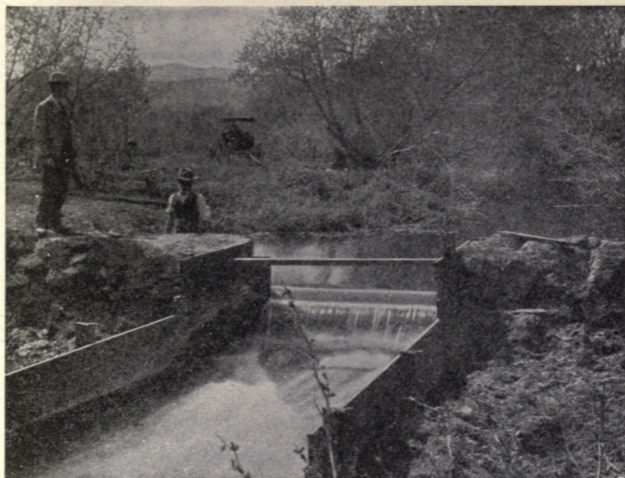
A. WEIR MEASUREMENTS OF LOS ANGELES RIVER IN SAN FERNANDO VALLEY, CALIFORNIA.
