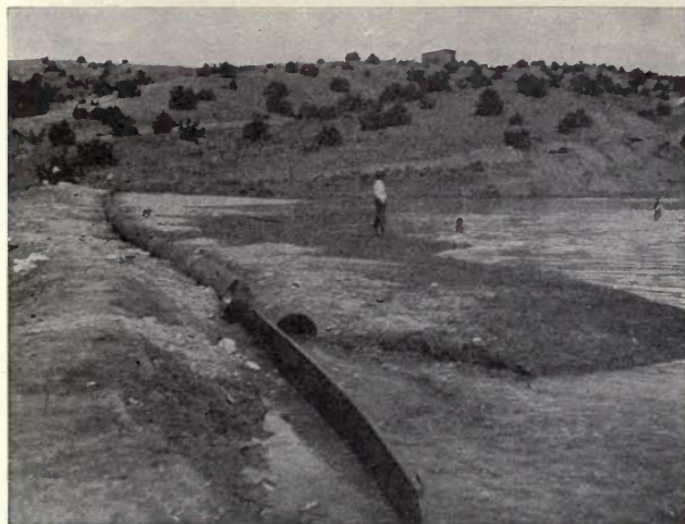
B. BUILDING DAM BY HYDRAULIC PROCESS AT SANTA FÉ, NEW MEXICO, SHOWING OUTLET PIPE.
