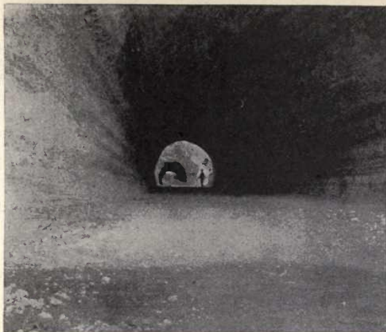
A. TUNNEL ON TURLOCK CANAL, CALIFORNIA.
