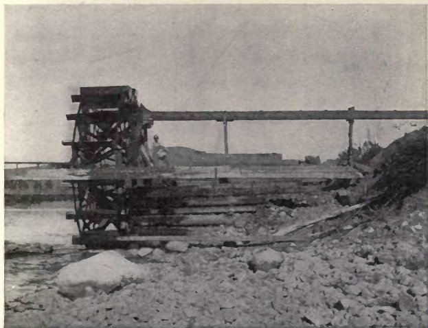
CURRENT WHEELS LIFTING WATER.
