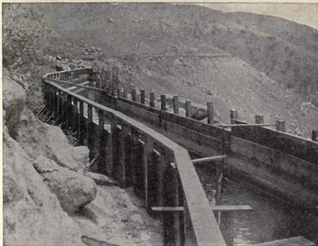
A. FLUME ON ROCKY HILLSIDE.
