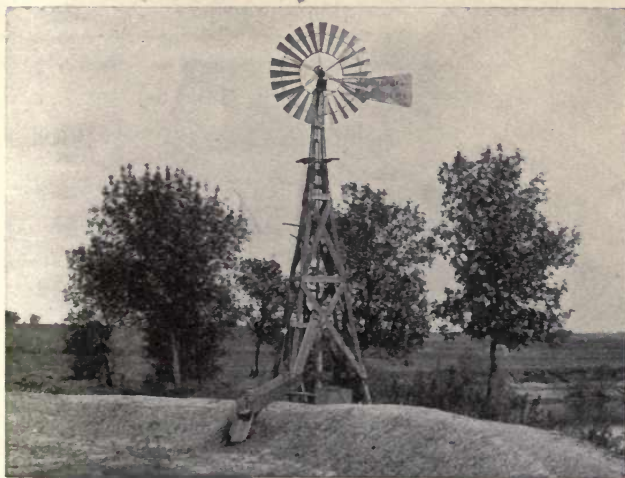
B. WATER FOR IRRIGATION PROVIDED BY WINDMILL.
