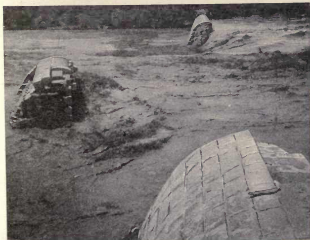
B. PORTIONS OF AUSTIN DAM IMMEDIATELY AFTER FAILURE.
