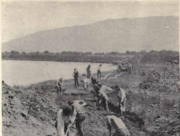
A. DIGGING A DITCH FROM A RIVER.
