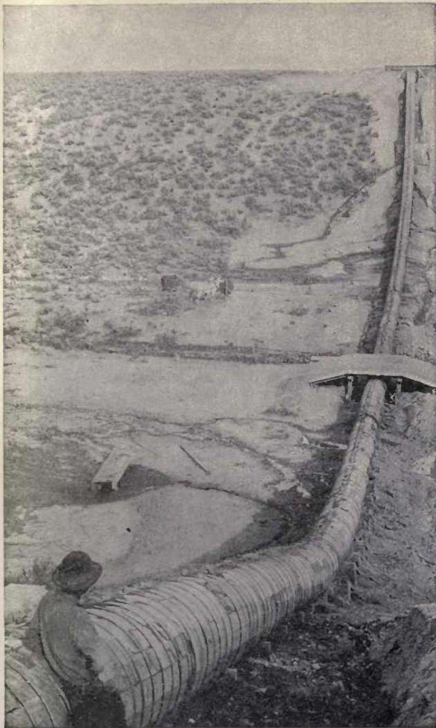
WOODEN PIPE LINE ON PHYLLIS CANAL, IDAHO.
