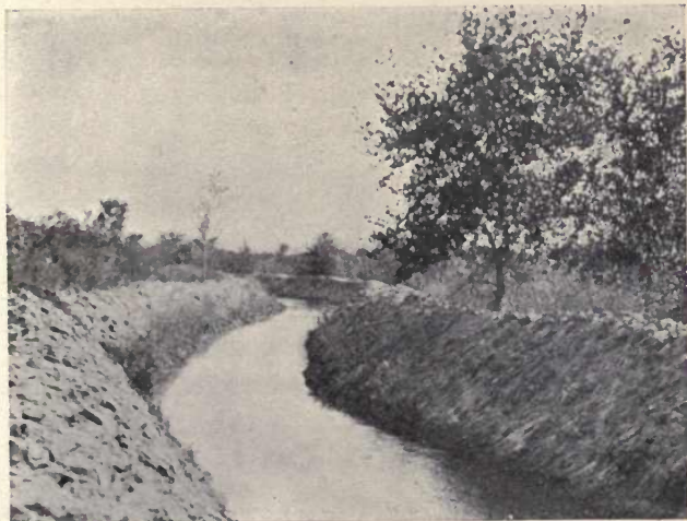
B. THE FINISHED DITCH.
