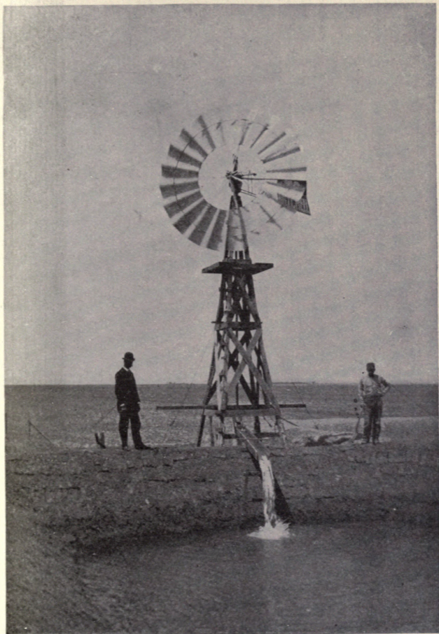
WINDMILL PUMPING INTO SOD-LINED RESERVOIR.
