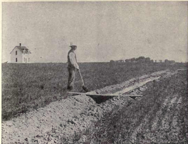
A. CANVAS DAM IN TEMPORARY DITCH.
