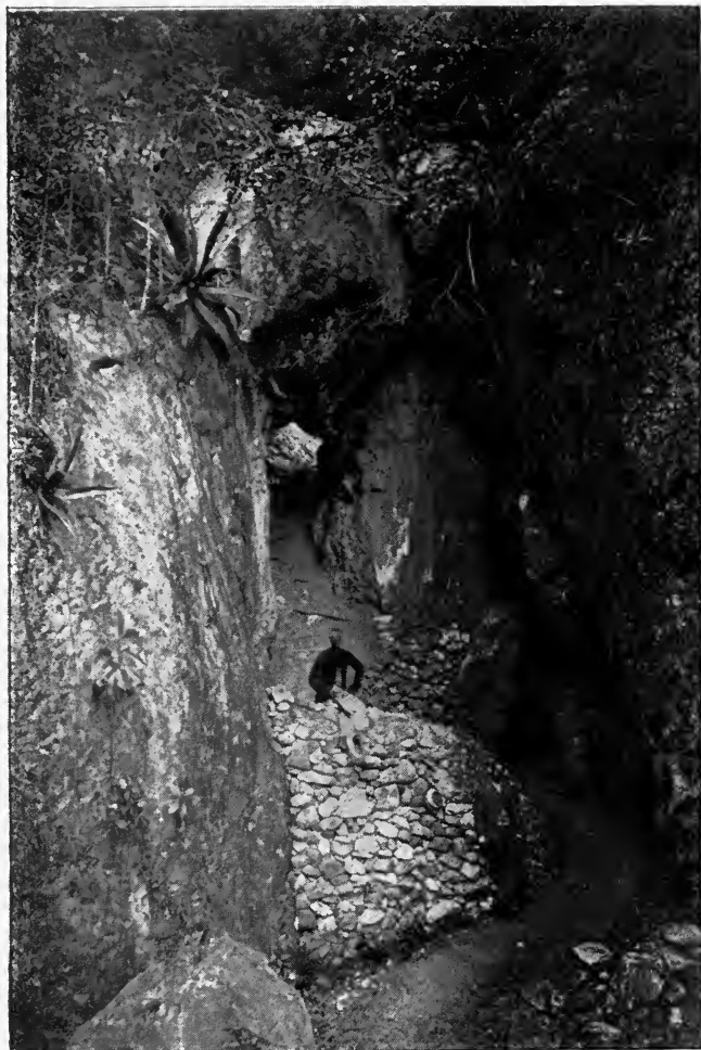
ROADWAY, CANE RIVER.
