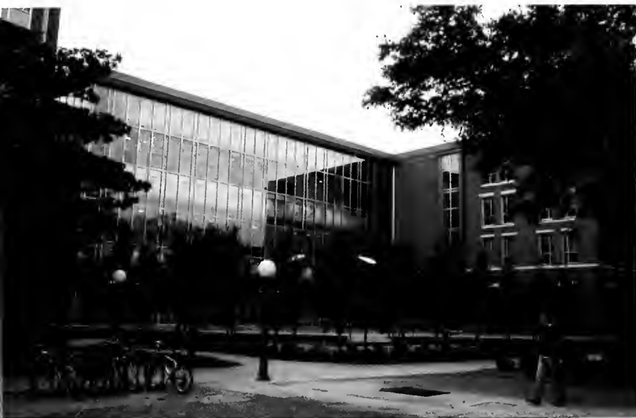
The back of Goldring/Woldenberg II, which features a $1.5 million trading room.
