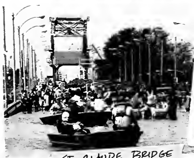
ST. CLAUDE BRIDGE August 30, 2005
