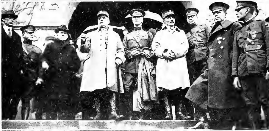
UPPER PICTURE: AT ATTENTION LOWER PICTURE: AT EASE
