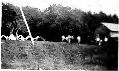
FLAG POLE ERECTION
