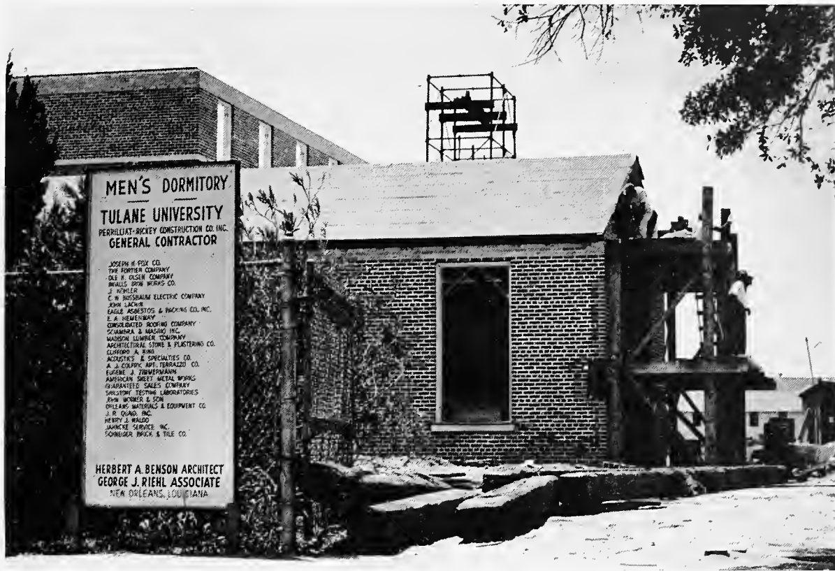
Samuel F. Zemurray Memorial Athletic Dormitory under construction
