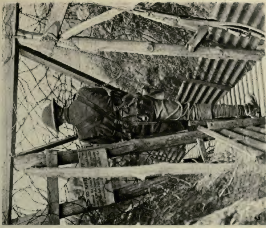
two flag-poles, and is sounded when warning is received of an impending gas-attack ; (2) A protection against trench-raids : the gate is lowered—like an ancient porticulis—when a raid is expected. As, in operations of this kind, speed is everything, the device has proved most successful.
