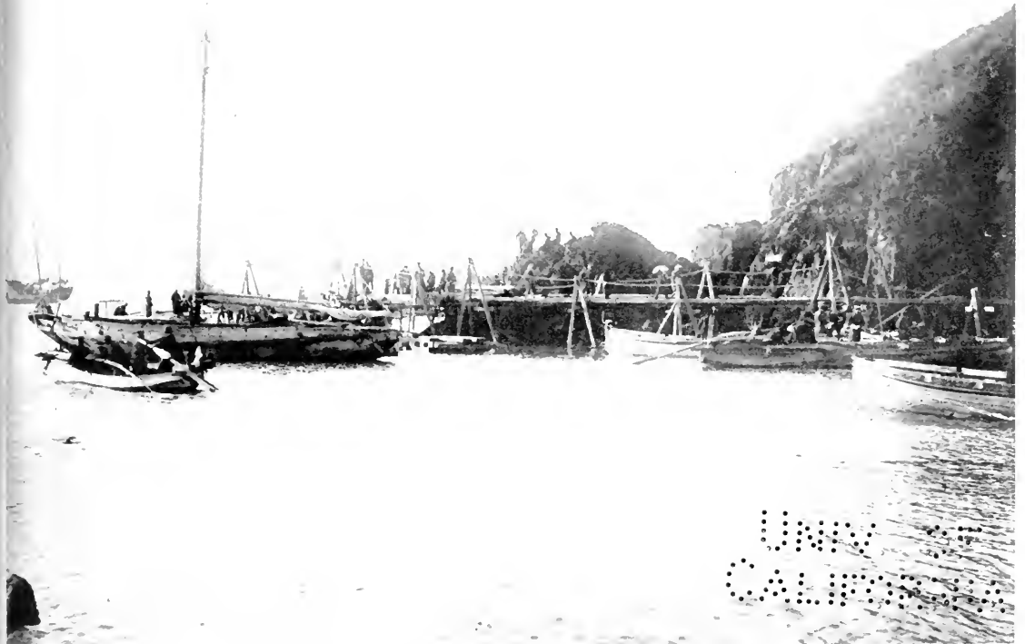
TEMPORARY PIER AT HWAYUAN-KOW AT FULL TIDE.
