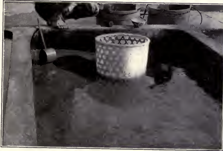
DRAWING DOWN A CONCRETE REARING POND
