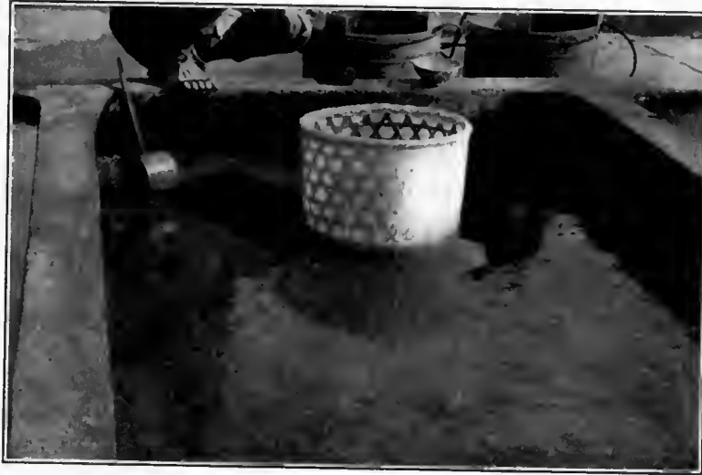
DRAWING DOWN A CONCRETE REARING POND
