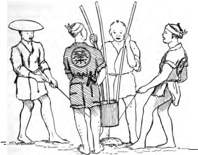
FIG. 5. — POUNDING DOWN FOUNDATION STONES.
