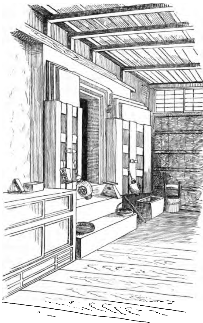
FIG. 139. — SPACE BETWEEN DWELLING AND KURA, ROOFED OVER AND UTILIZED AS A KITCHEN IN TOKIO.
