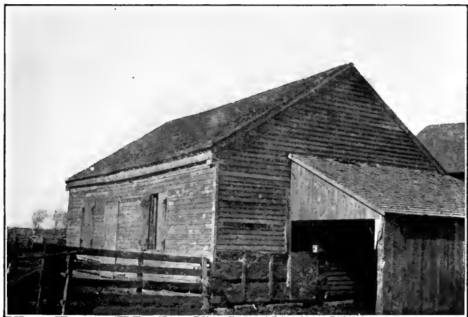
OLD LOG CHURCH, BUILT ABOUT SIXTY YEARS AGO The hewn logs are now covered with boards
