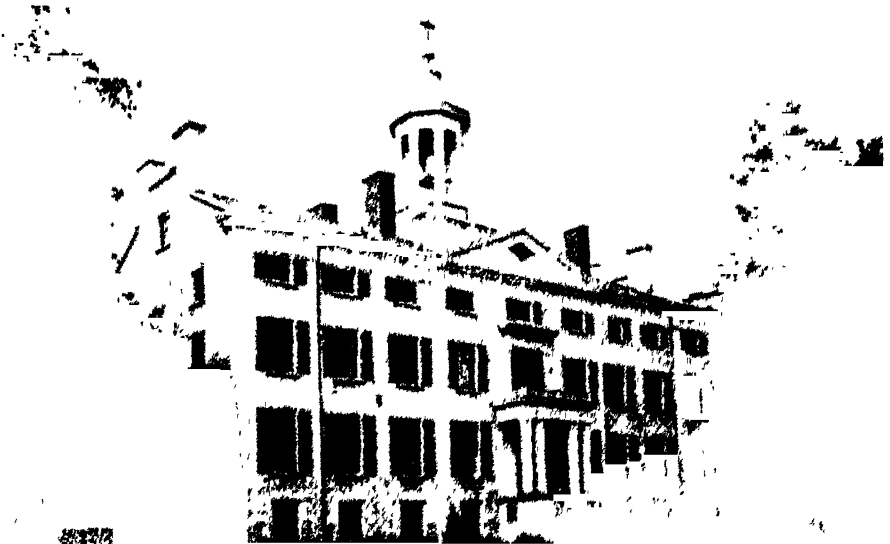
The "Rock Building," St. Stanislaus Seminary, Florissant A dignified structure of fortress-like solidity dating from the forties. Built of Missouri lime-stone from near-by quarries, its walls being lined with thicknesses of brick made on the premises by the hands of novices.
