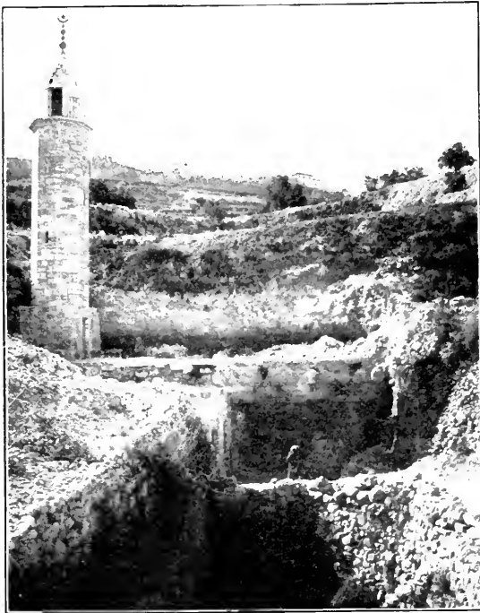
THE POOL OF SILOAM
