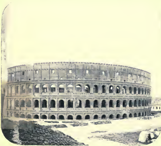
THE PRESERVED WALL.
