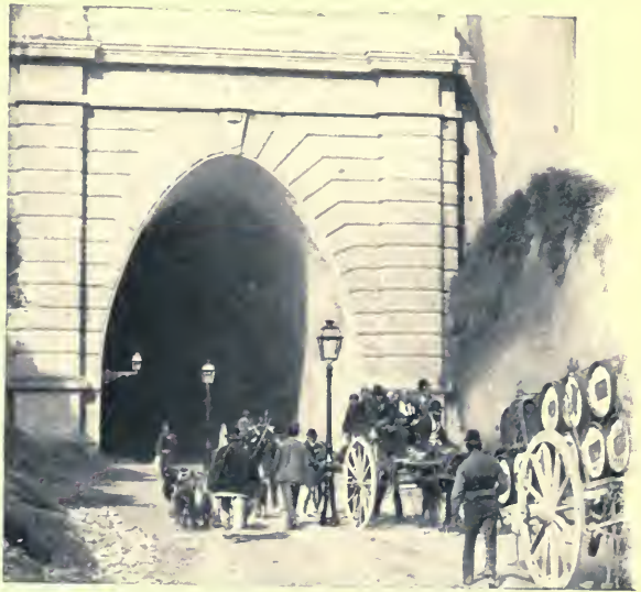
THE NEW TUNNEL.
