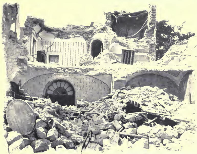
DRAWING-ROOM OF LA PICCOLA, AFTER THE EARTHQUAKE.
