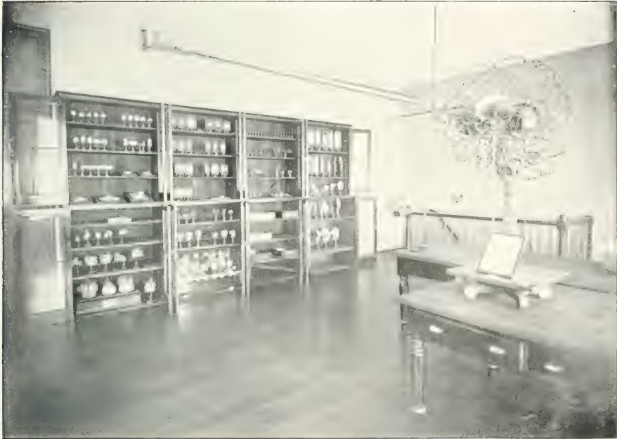
FIG. 12. NORTHWEST CORNER OF THE STUDY ROOM ON THE THIRD FLOOR.
