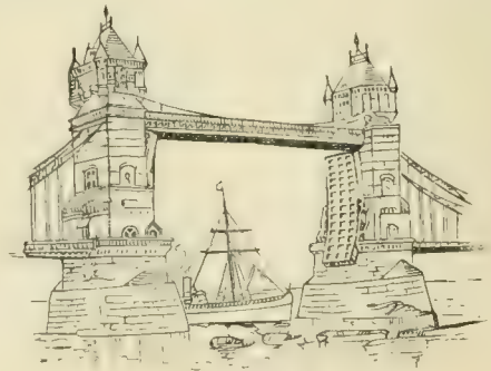
Tower bridge, London, England.
