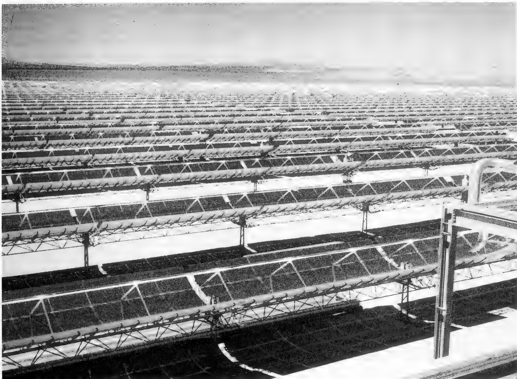
Fig. 1. Photo of Luz plant in California, taken by the author.
