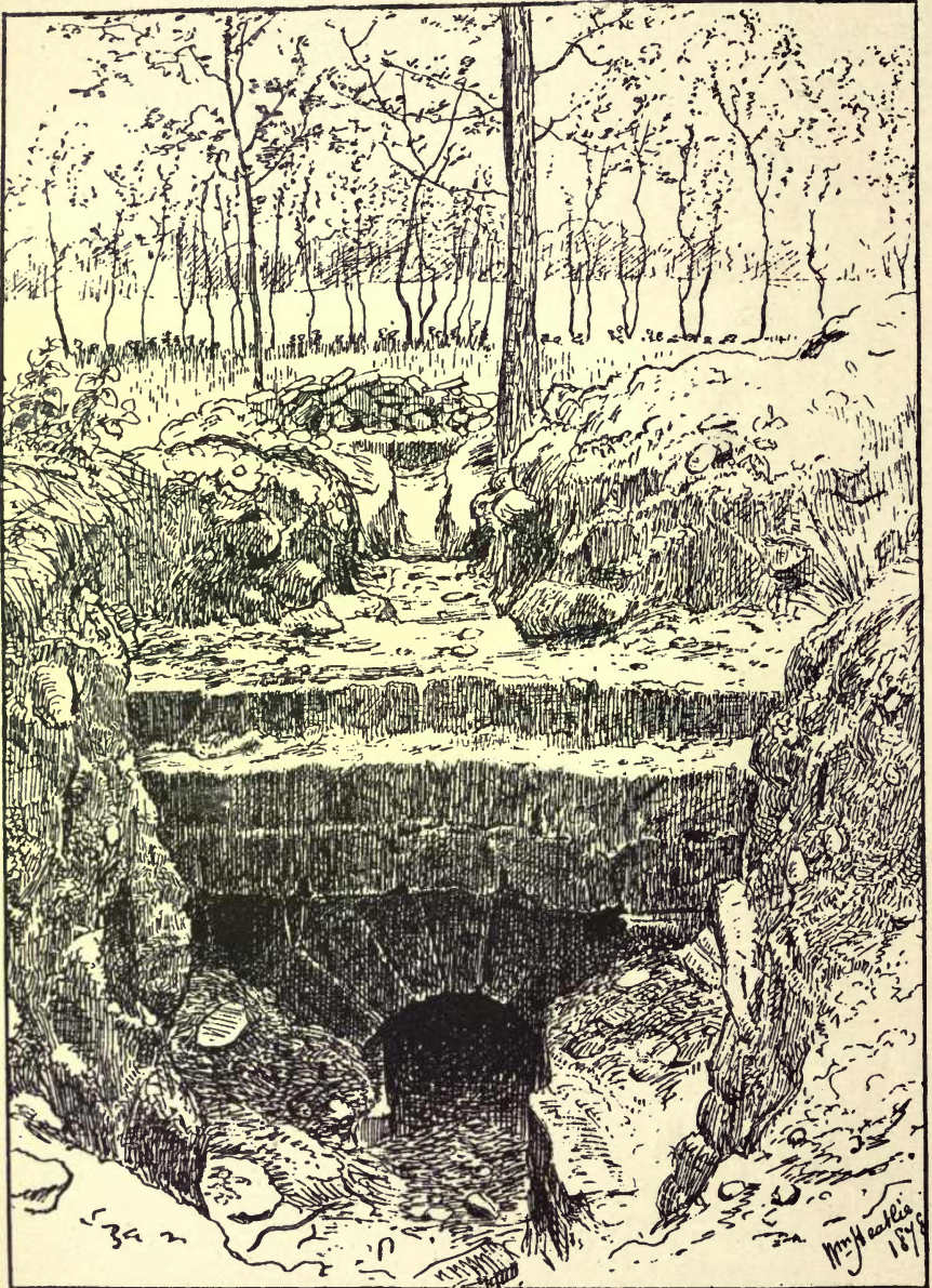
RAMPART AT NORTH-EAST CORNER, WITH CULVERT (INNER FACE).
