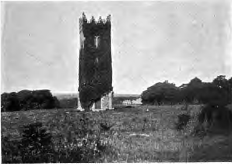
"THE STEEPLE," OR "THE TOWER," AT CARTON.
