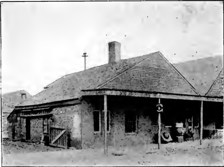
Building in which Stephen A. Douglas taught school. Winchester, Illinois.
