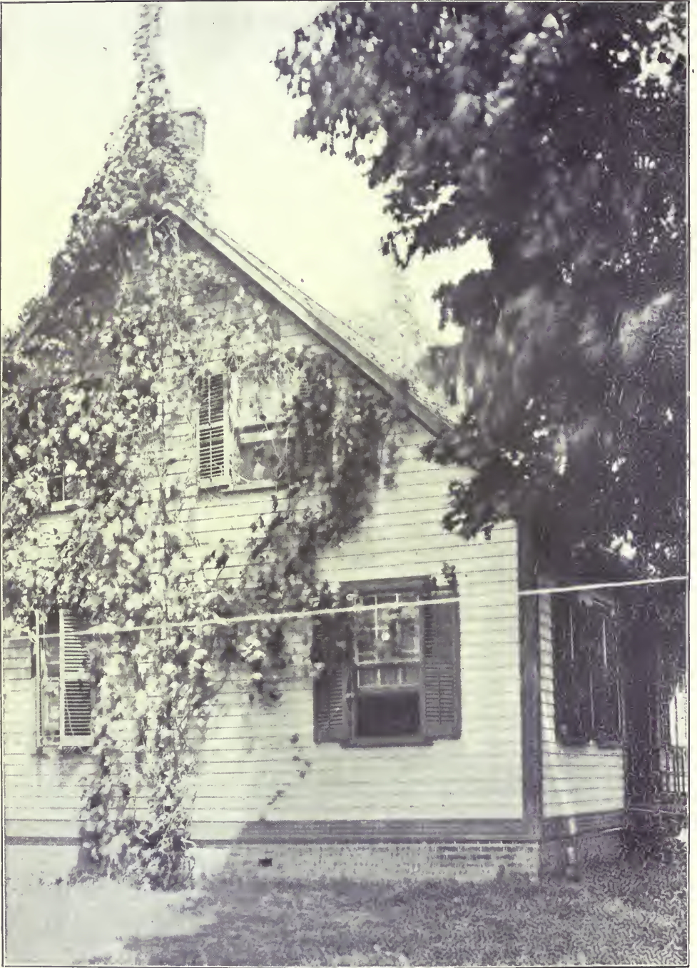
West End of Reid House on Homestead Farm.
