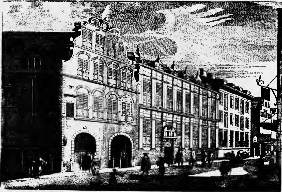
BUILDING OF THE DUTCH EAST INDIA COMPANY IN AMSTERDAM, HOLLAND Through this great trading organization much of the Dutch colonization of New Netherland was effected.
