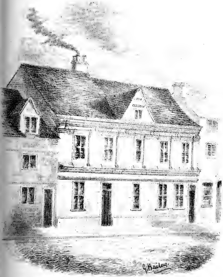
Old house in Walker Lane.
