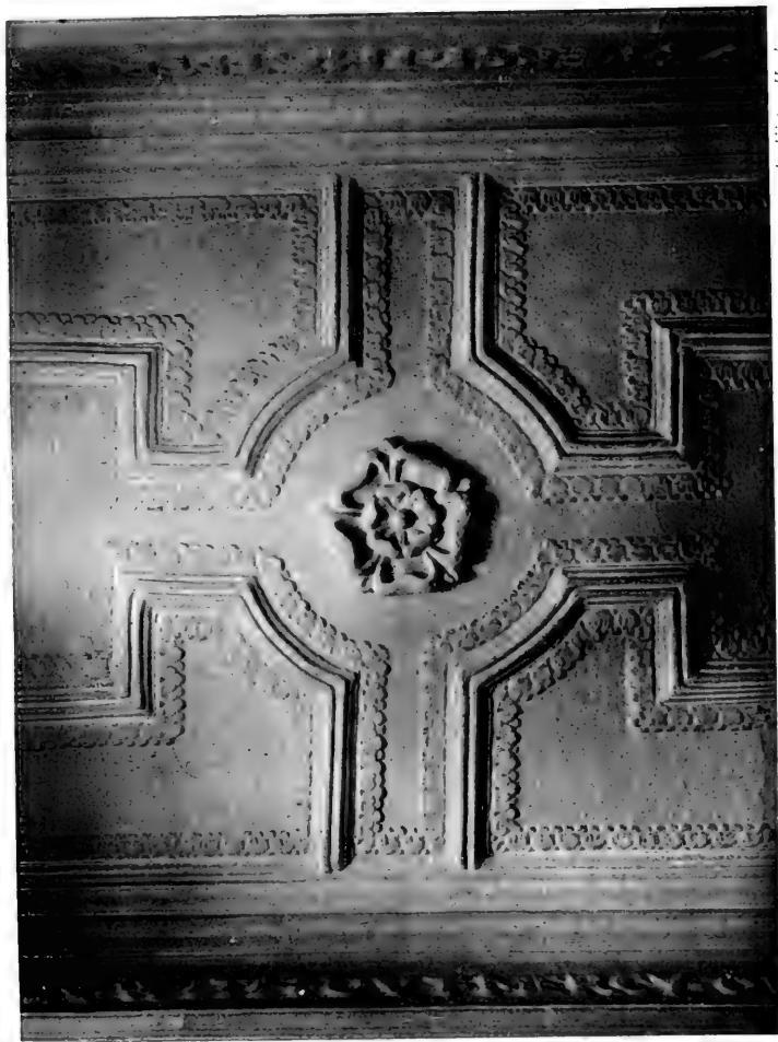
BRADSHAW HALL, CEILING OVER THE STAIRCASE.
