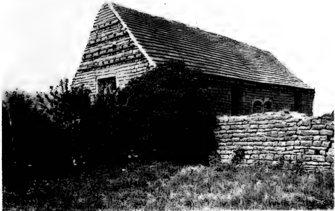
PADLEY HALL (FROM THE NORTH-EAST).
