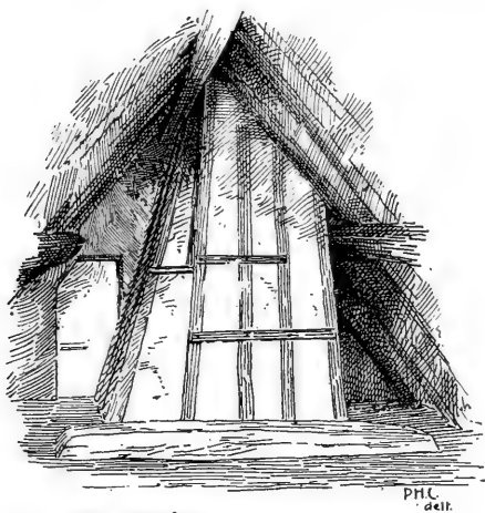
THE CHIMNEY IN THE ATTIC SOUTH SITCH
