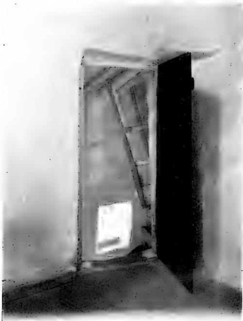
TOP OF STAIR IN UNDIVIDED HOUSE.
