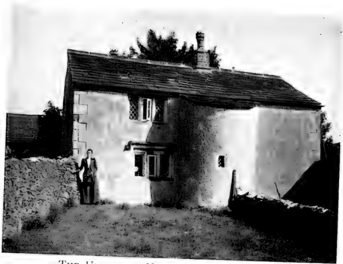
THE UNDIVIDED HOUSE (FROM THE SOUTH).
