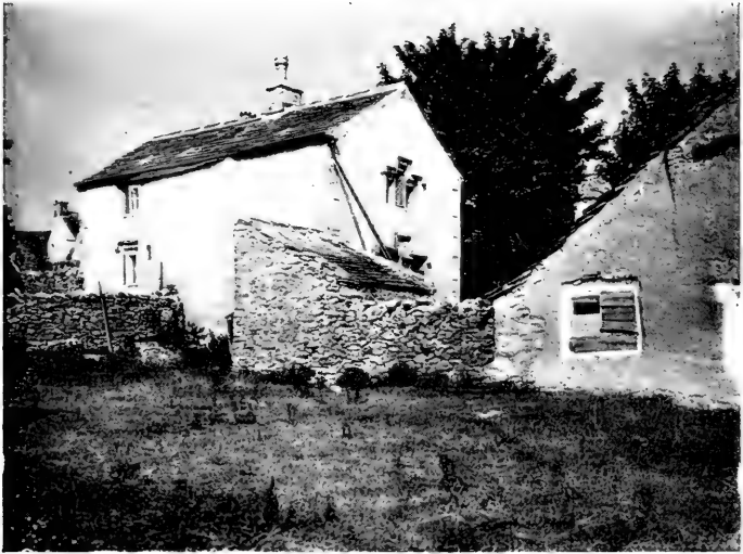
HOUSE AT LITTLE HUCKLOW (FROM THE SOUTH).
