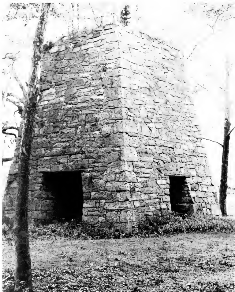
Figure 5. Zane's first furnace, later the A. P. Taylor Furnace, located on Furnace Run in Frederick County, Virginia.
