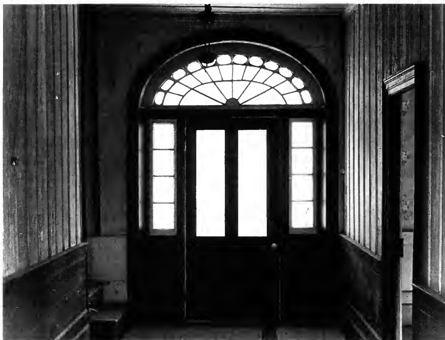
6. Fan-lighted front door from interior, before restoration. Photograph courtesy of the Murfreesboro Historical Association, Inc.
