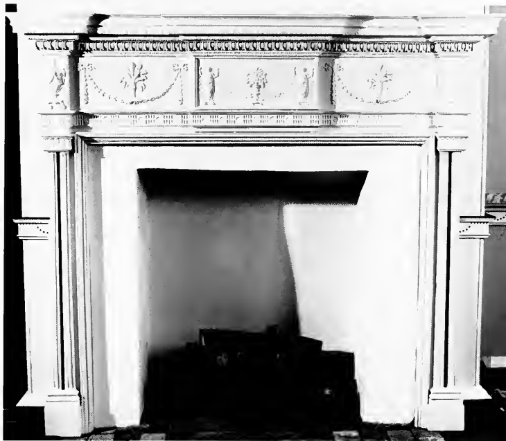
28. Mantel with composition ornament by the firm of Zane, Chapman & Wellford. John Steele House, Salisbury, North Carolina, 1800. HOA 65 \frac{3}{8} ", WOA 74 \frac{1}{4} ". MRF 27,286.
