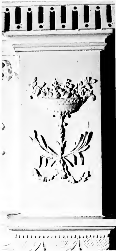
27. Truss block of a mantel with composition ornament by Robert Wellford, floral decoration, 1806. HOA 9", WOA 4 1/2". Jacob Miller House, near Lancaster, Pennsylvania. Photograph by the author.
